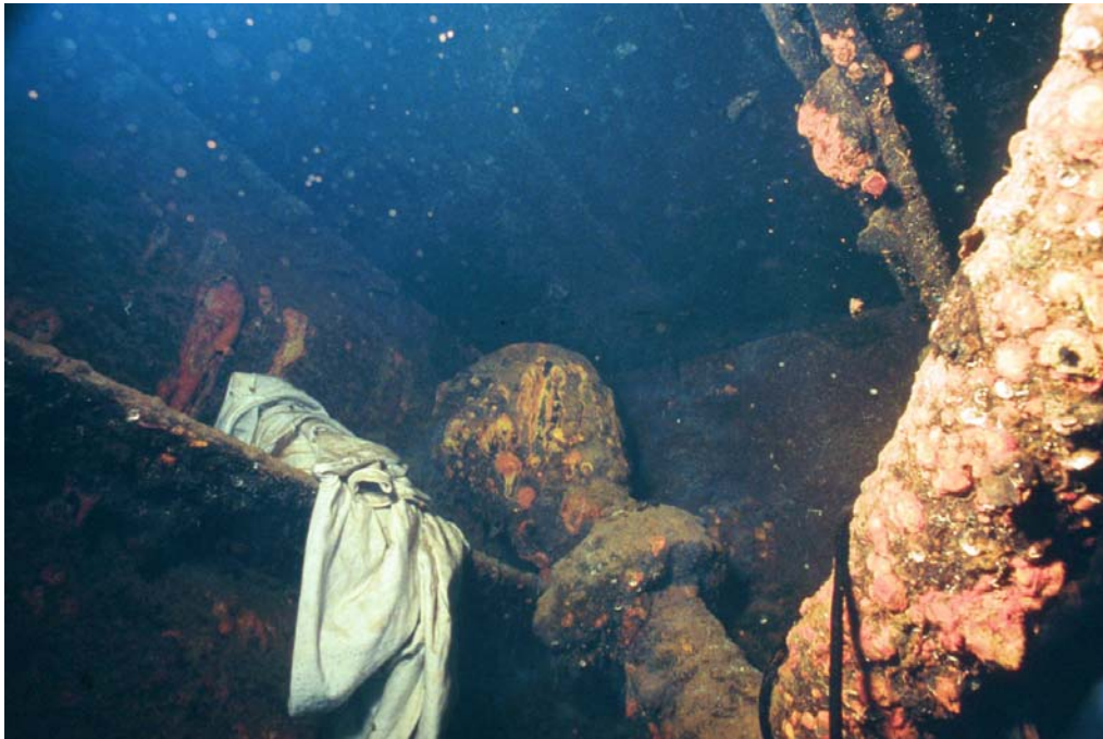
Figure 4. COT 4-S, Bellmouth Oil Leak Source
