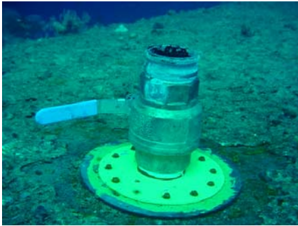
Figure 4-12. Valve Threaded onto Flange
