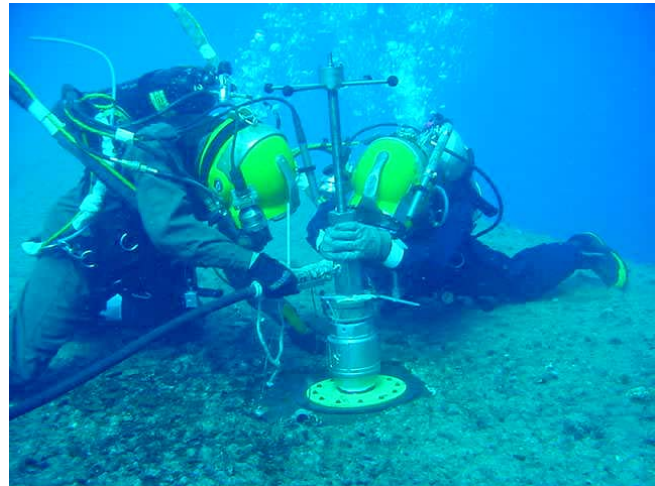
Figure 4-8. Two Divers Working the Hot Tap Machine on Mississinewa 's Hull
