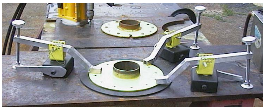
Figure 4-10. Hot Tap Flange Held in Place with Magnets
