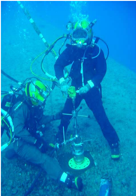
Figure 4-13. Two Divers Drilling into Mississinewa's Hull with a Hot Tap Machine
