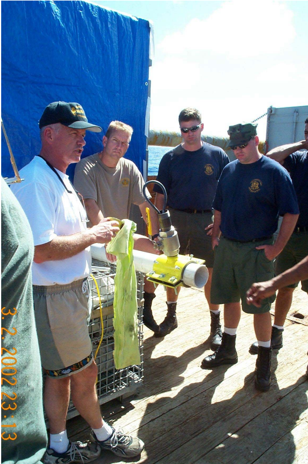
Figure 17. Enroute Training: Balloon Pipe Stopper Through Hot Tap Hole
