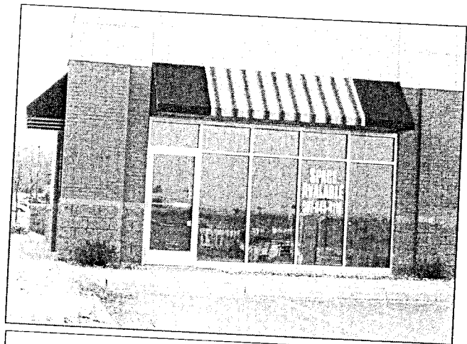
Site of new facility intended to serve the Northfield Underserved Area beginning Summer 2004.
