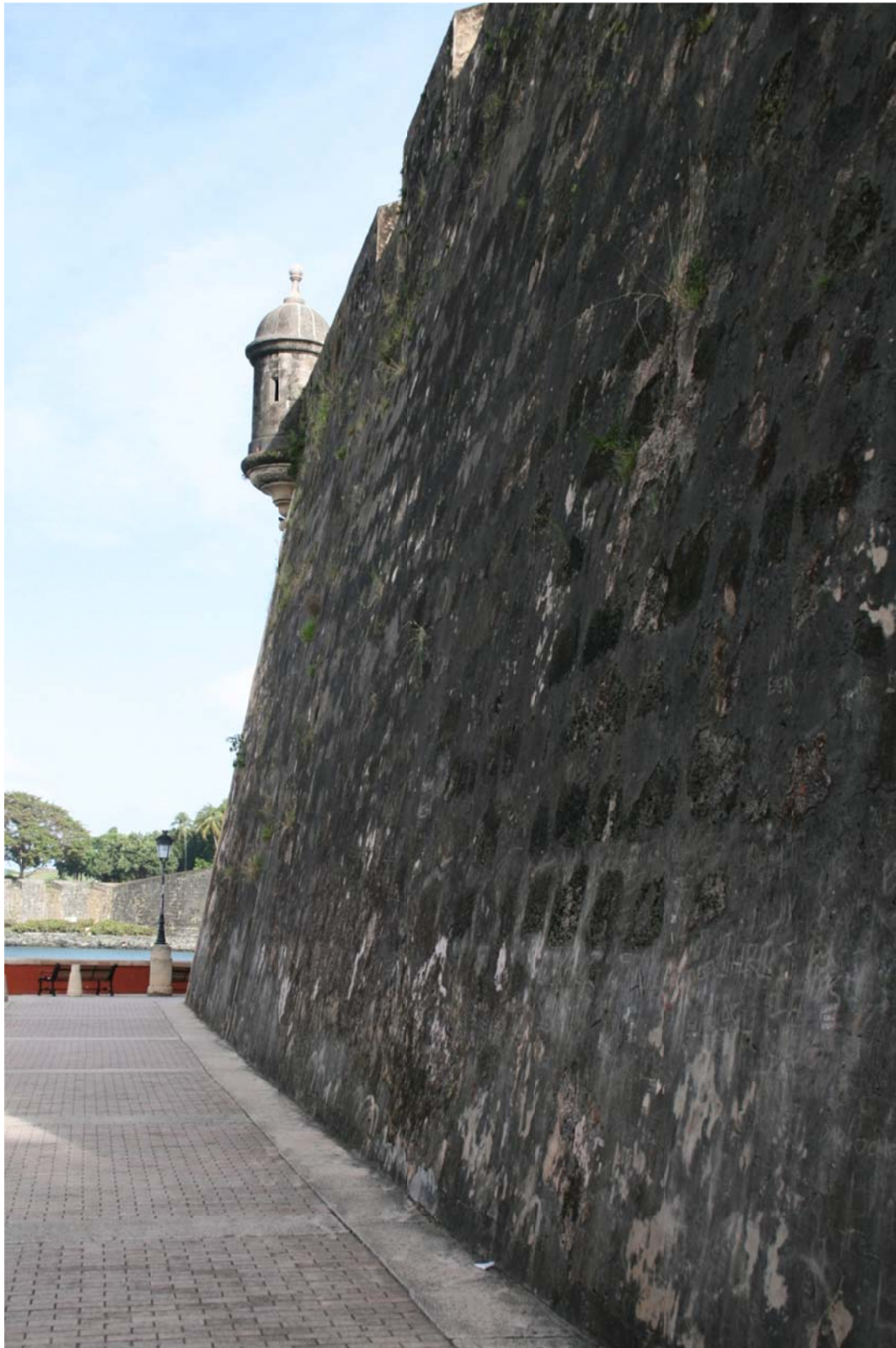
South Wall, south façade, camera facing north.
