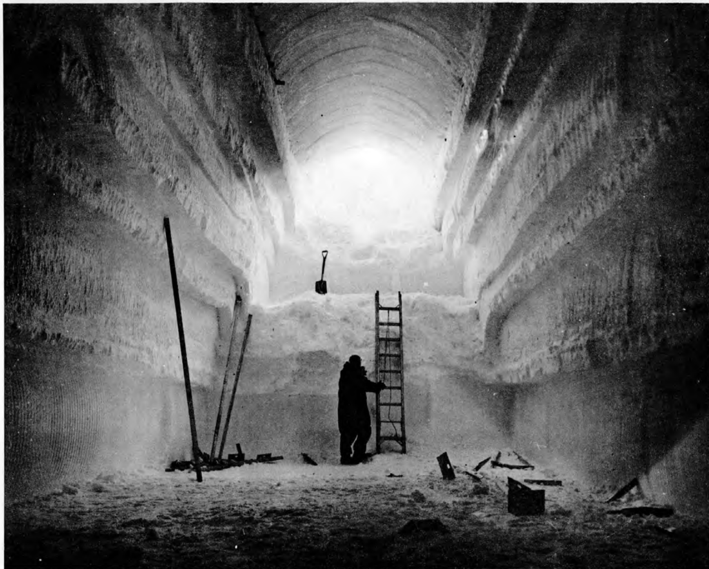
Figure 15. Unsupported snow arch after metal forms have been removed.
