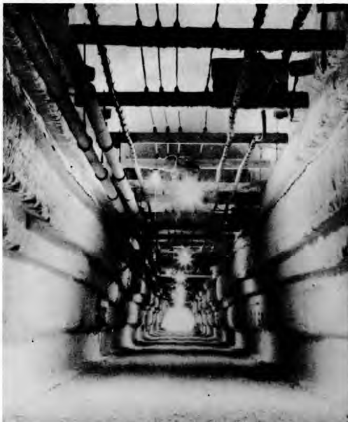
Figure 36. View of main communication trench showing overhead utility lines.
