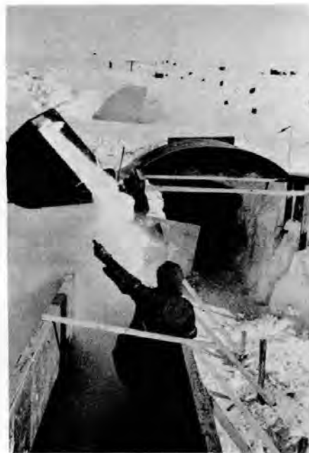
Figure B2. Traxcavator filling plywood forms with Peter-miller snow.
