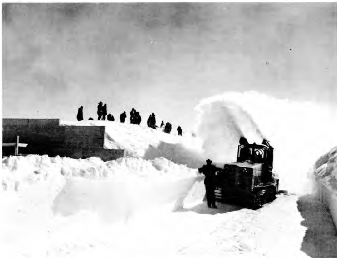
Figure 7. Peter snow miller in operation cutting a trench.
