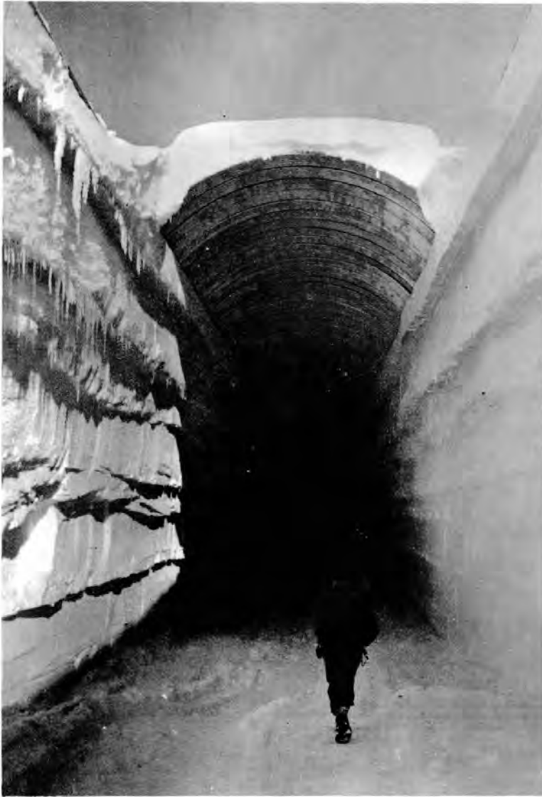
Figure 11. Undercut trench.
