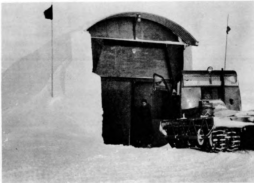
Figure B4. Vehicular access door.
