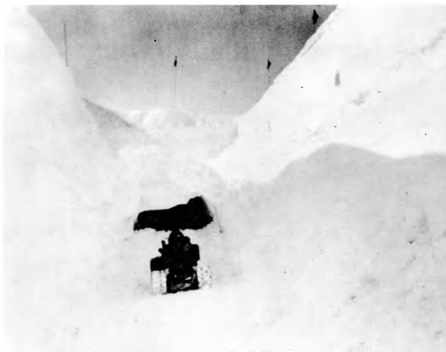
Figure 17. View of portal to Camp Century showing dozer clearing snowdrifts after a storm.
