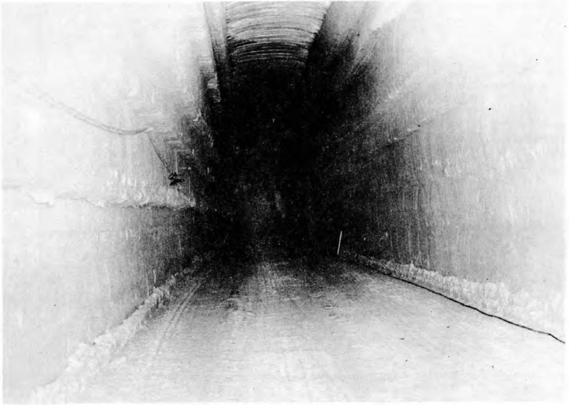
Figure 2. Snow tunnel (cut-and-cover type).
