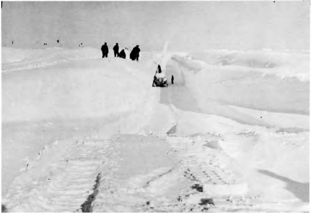
Figure 9. Peter miller cutting a straight-wall trench.
