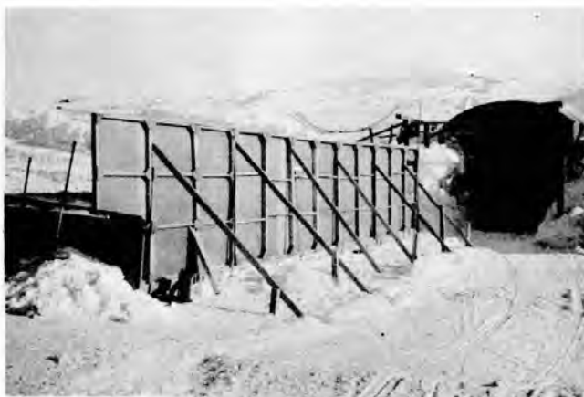
Figure B1. Erection of 14-ft high plywood forms.
