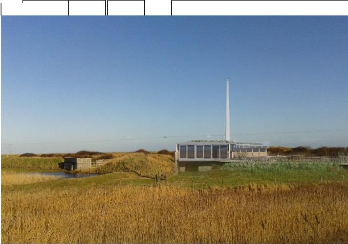
Proposed View Looking onto Site from Flood Bank Path
