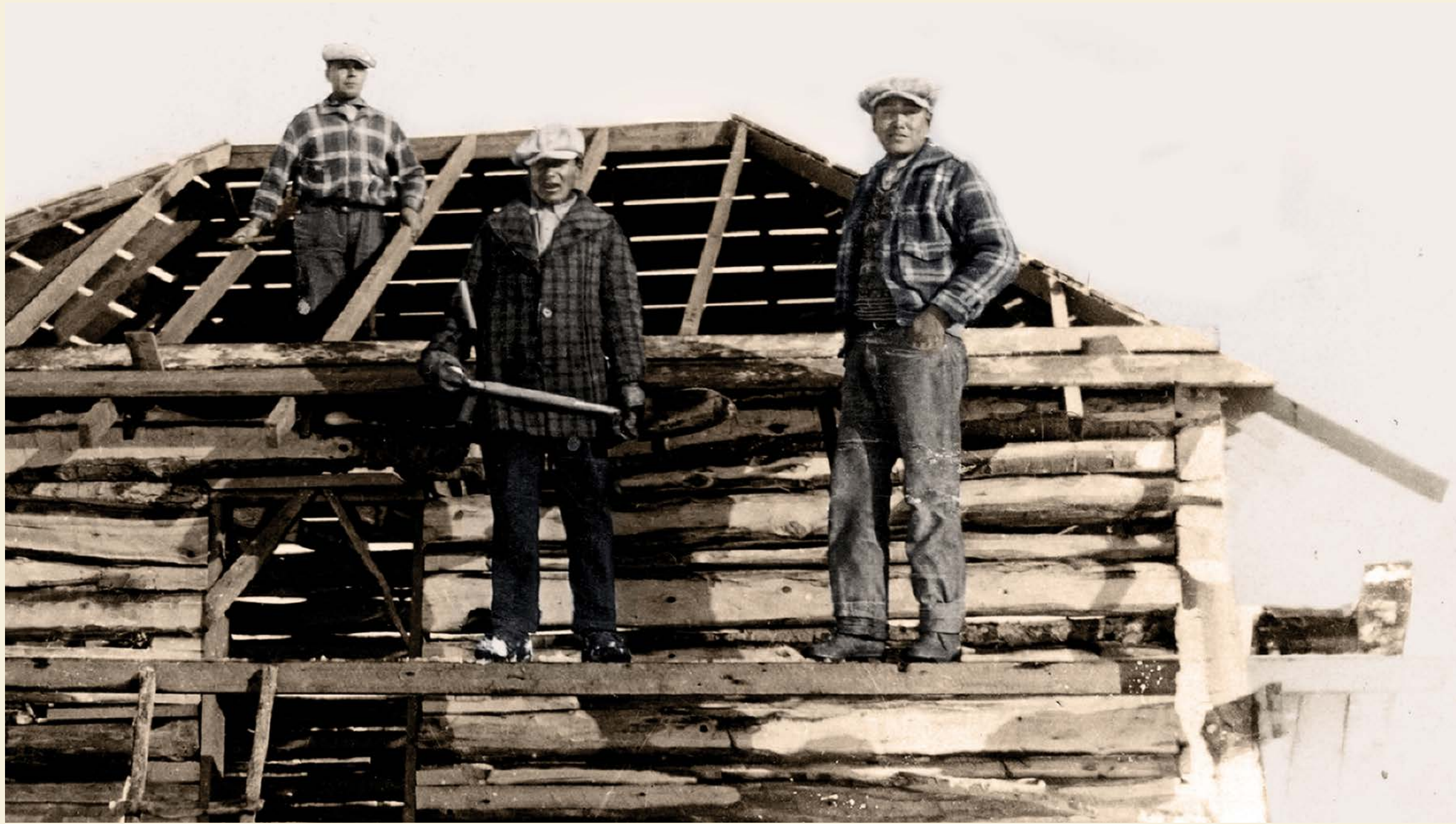
William Littlecrow, Jimmie Littlecrow, and William Eagle building a log house. Through the mid-twentieth century, people of Whitecap Dakota First Nation built their own homes on the reserve, or would volunteer to build homes for those who could not build their own. They were made of logs that were filled with the combination of fine hay and plaster. They would re-plaster the houses every year.
