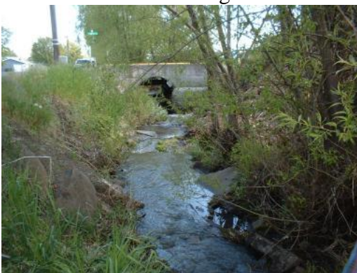
Photo 10. Site #8 looking downstream. (May 2010).
