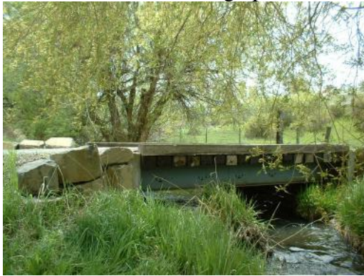
Photo 15. Site #5 looking upstream.
