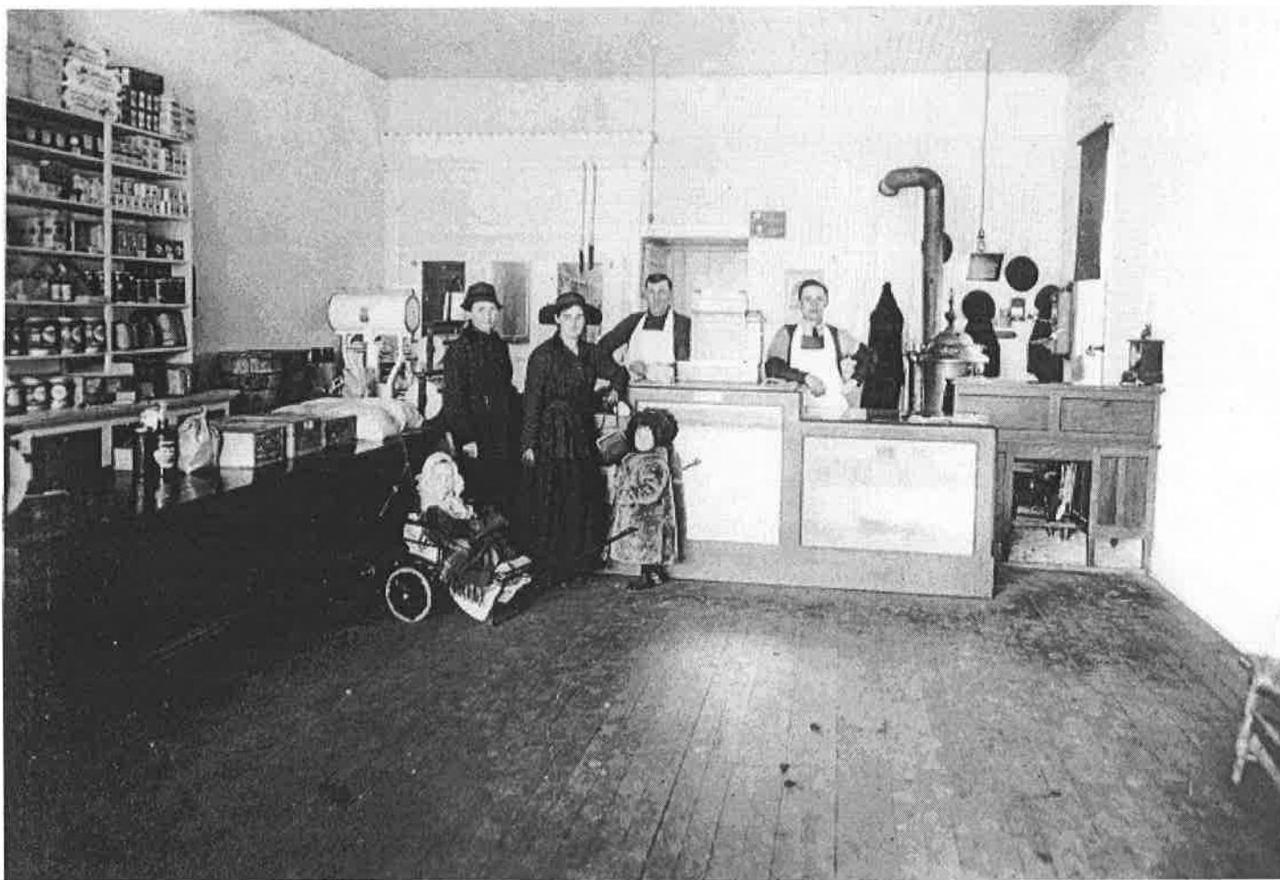
Figure 8: The interior of this grocery store in Sheffield, Iowa, photographed in February 1920, is not unlike the layout of the store at 518 E. Bowery. On the right side of the photo, the stovepipe from a pot belly stove helps heat the room before venting through a hole in the fireplace. A refrigerated meat locker, cooled by blocks of ice, can be seen in the left back corner. Large windows at the front of the store provide illumination. Original in Special Collections, State Historical Society of Iowa, Iowa City.
