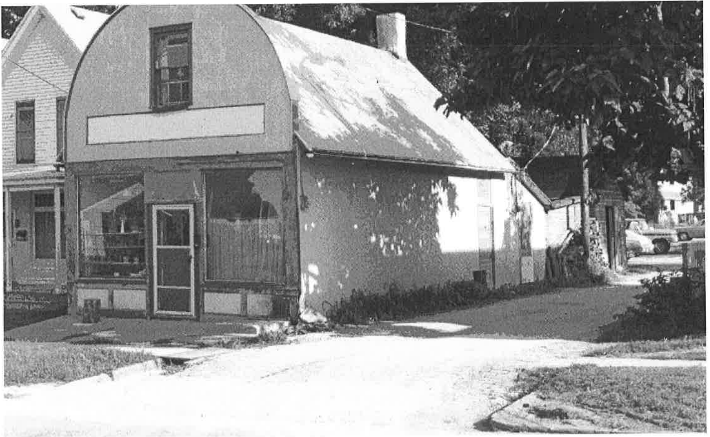
Figure 1: Exterior of 518 E. Bowery in about 1982. Original color slide owned by Richard Hugill. The false front created the illusion of a larger store, while hiding the gable roof line. Typically, a sign appeared on the upper façade and large display windows facing the street showcased products for sale, thus enticing customers into the store.
