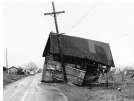
Heavy runoff floated a barn roadside in the Umpqua River Basin.
