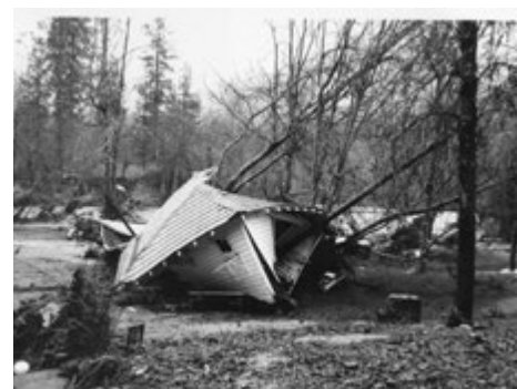
Raging water in the Rogue River Basin moved houses downstream of their foundations.
