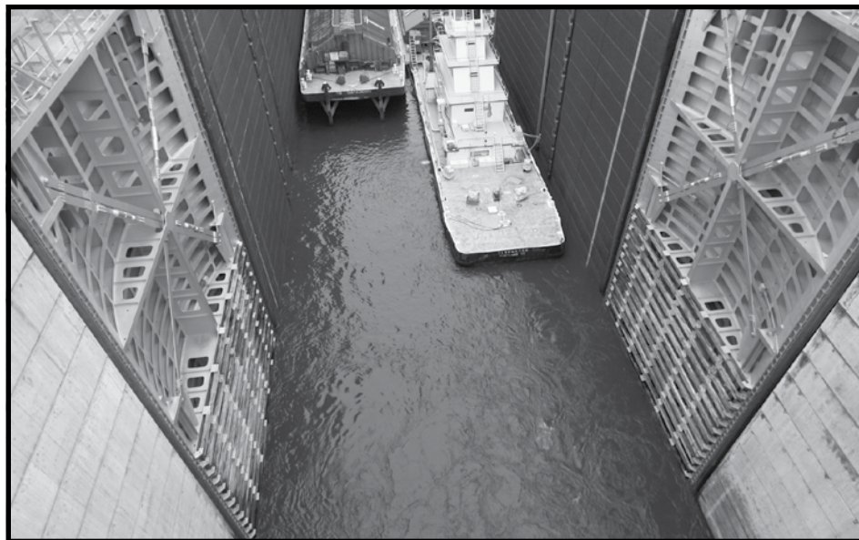
The twin gates at The Dalles navigation lock are typical of the huge yet functional structures at many Portland District projects that support the nation’s infrastructure and economy.
