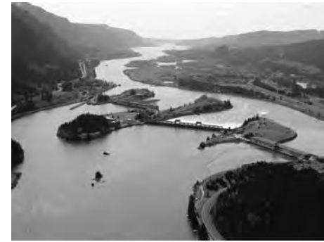
Bonneville Lock and Dam is located about 40 miles east of Portland, Ore.
