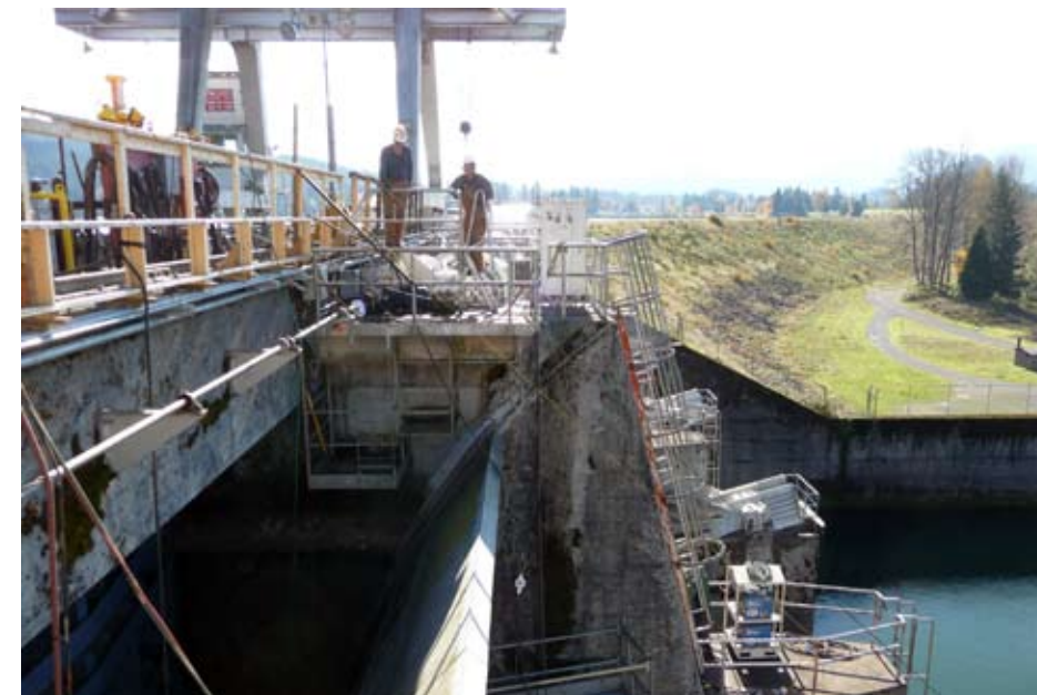
Dexter Dam’s seven spillway gates have been rehabilitated and the IRRMs limiting reservoir levels to below the upper struts have been lifted.
