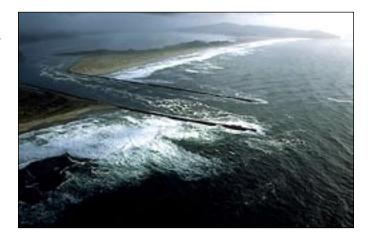
The 5,700-foot-long north jetty was constructed in 1933, rehabilitated in 1965, and again in 1991. In 1965, construction of a south jetty 8,000 feet long was authorized. Work began in 1969 and the first segment was finished in 1971. Construction of the second segment was completed in 1974. Construction of the third segment— 1,500 feet to complete the 8,000-foot jetty started in 1978 and was completed in 1979.
