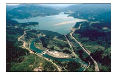
lating outlet tunnel, power penstock, and intake tower with multi-level intakes are located in the dam's right abutment; a gate-controlled concrete chute spillway is located in the left abutment. The powerhouse has a generating capacity of 49,000 kilowatts.
