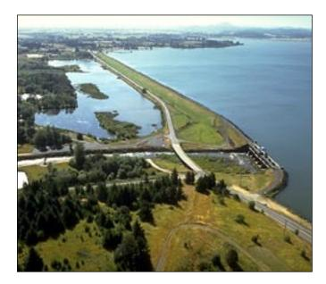
The Fern Ridge project, at River Mile 23.6 of the Long Tom River, is about 12 miles west of Eugene. The dam and reservoir have been in continuous operation since 1941. To provide for additional flood storage capacity, it was raised from 47 to 49 feet in 1965. The reservoir provides 110,000 acre-feet of usable flood control storage and controls runoff from a 275 square-mile drainage area, including the Amazon Creek Basin.
