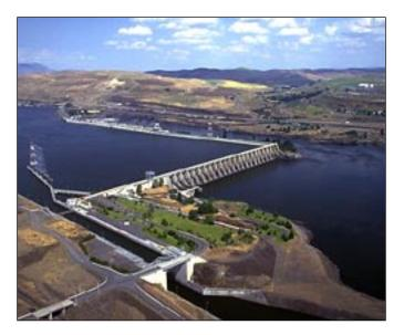
past the tumultuous rapids in that reach of the Columbia. Now the lake provides slack-water navigation at a minimum depth of 15 feet in the main channel. The project's navigation lock, on the Washington shore, is 86 feet wide and 675 feet long. It has an 88-foot normal lift and provides a 15-foot minimum depth over the sills. Waterborne traffic through the lock in 1999 was 8,670,000 tons.
