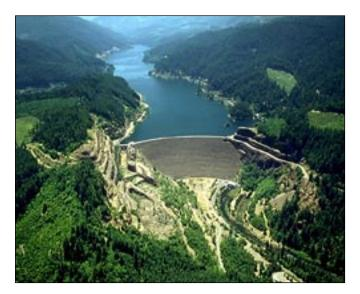
Cougar Lake has a storage capacity of 219,000 acre-feet and controls runoff from an area of 208 square miles. The lake's surface area is 1,235 acres at full pool. The dam rises 445 feet above the streambed.
