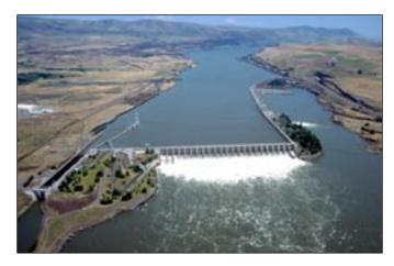
Navigation. Lake Umatilla provides slack water for navigation, with a minimum 15-foot depth in the main channel. The navigation lock, located on the Washington shore, is 86 feet wide, 669 feet long, and provides 15 feet of water depth over the sills. With a 113-foot maximum lift, it is one of the highest single-lift locks in the world. Lock traffic in 1999 was 8,259,000 tons.
