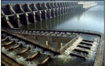
Mitigation Program, contracts were awarded in 1996 for a new fish passage system and flow deflectors. The fish passage system will include a 1,200-foot-long, five-footwide, 20-foot-deep chute extending along the Oregon shore from the powerhouse to the dewatering building. From the dewatering building, the young fish will travel through a three-foot-diameter flume to the sampling and monitoring building. After being monitored, the fish will be returned to the river downstream of the power-
