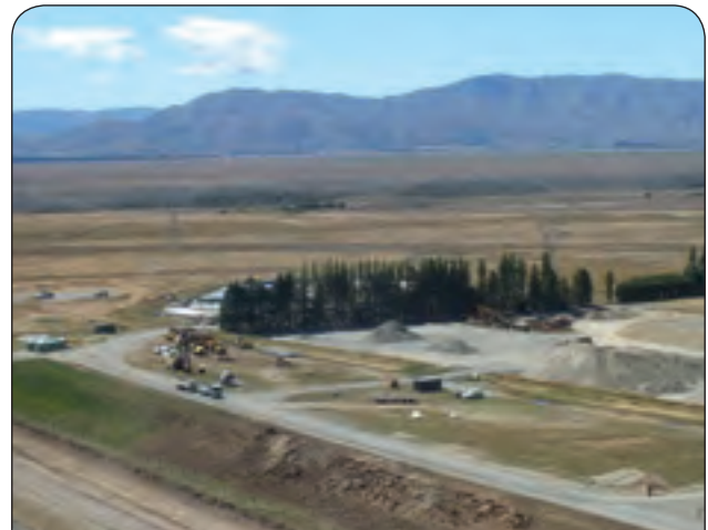
FIGURE 14 // Construction Management Site for the Tekapo Canal Remediation Project.
