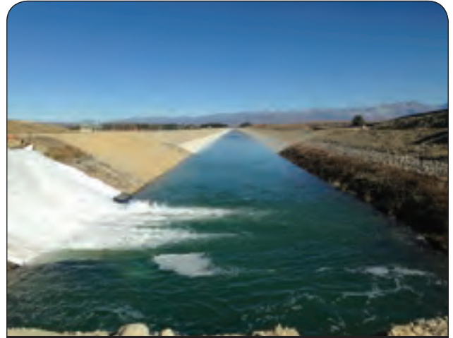
FIGURE 20 // Re-watering a repaired section of the Tekapo Canal.
