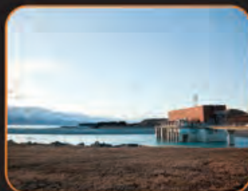
TEKAPO B POWER STATION Two 80 MW Units. Commissioned 1977
