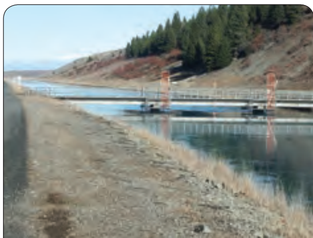
FIGURE 25 // No. 1 Farm Bridge undergoing seismic strengthening works.
