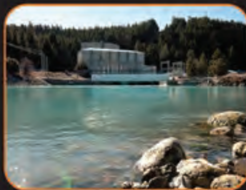
TEKAPO A POWER STATION One 25 MW Unit. Commissioned 1951
