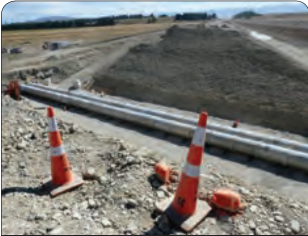
FIGURE 22 // 8.17 km culvert pipes being installed.
