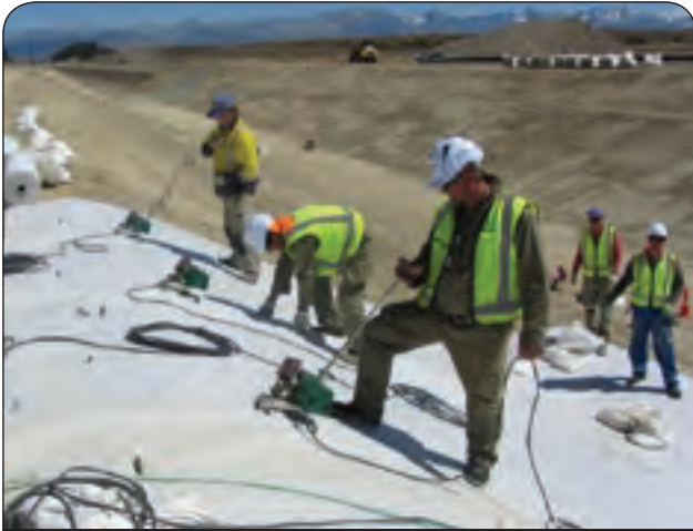
FIGURE 18 // Welding equipment joining sections of liner together.
