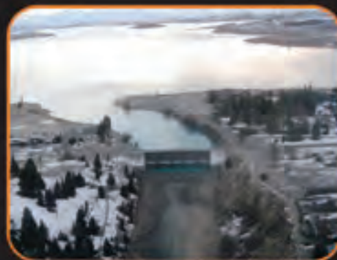
LAKE TEKAPO CONTROL STRUCTURE (Gate 16)
