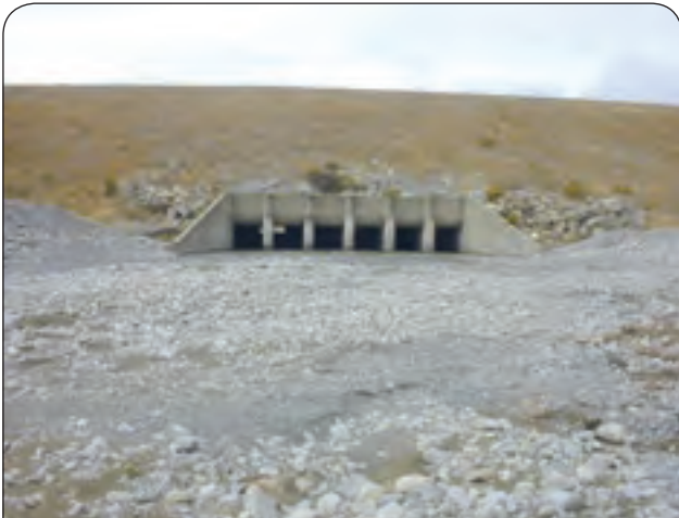
FIGURE 38 // Fork Stream culvert clear of debris following maintenance works.
