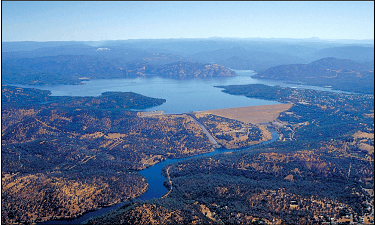
Figure 1. Oroville Dam, Powerhouse, and Spillways. Ungated spillway lip is the lengthy low point to the left of the main service spillway. Regulated design-release out flows of up to 150,000 cfs could flow downslope across the hillside during Corps of Engineers required surcharge operations.
