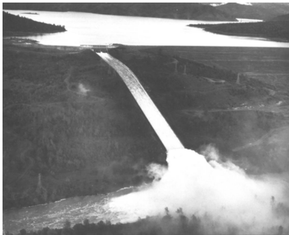
Figure 5. 1986 main service spillway operations. Note the ungated spillway to the left, and transmission line towers and road downstream. ACE required design-outflow surcharge operations call for an operational regulated release that could deliver up to this flow over the hillside, reducing and eventually shutting down flows in the service spillway. DWR
