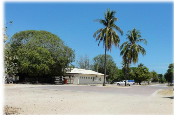
Figure 12 – Pormpuraaw Council Building near Central Park
