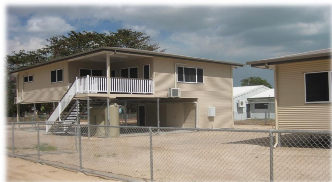
Figure 7 – One example of new Housing in Pormpuraaw
