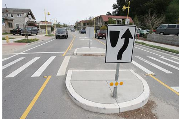
Photo of Pedestrian Refuge Island (note that detectable warning surface should be provided on either edge of the opening in the island).
