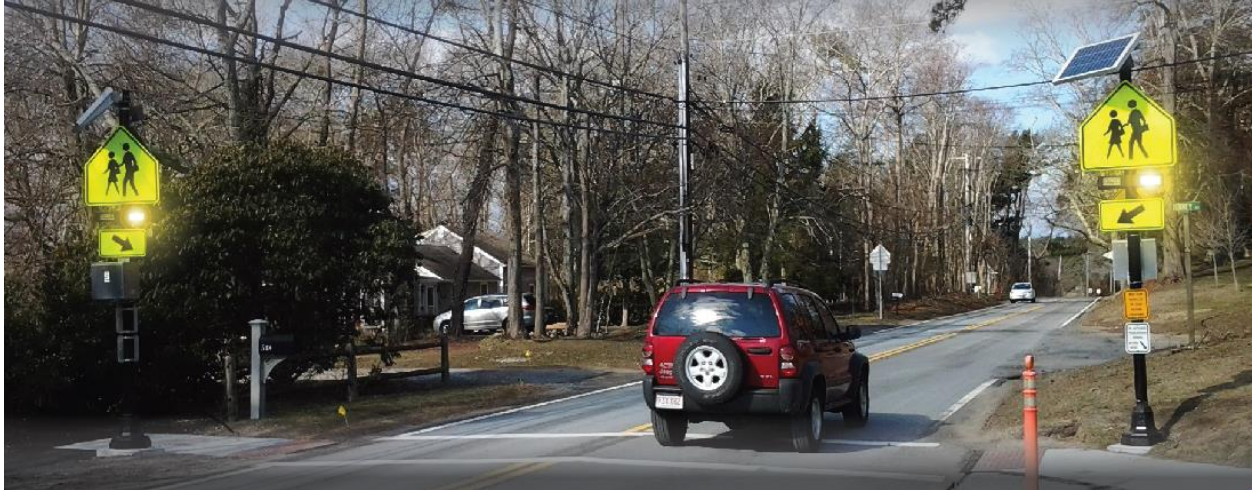
Figure 1 - Gate-posted RRFB installation at a school crosswalk
