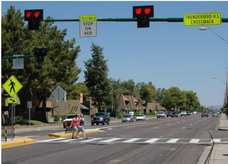
Typical installation of Pedestrian Hybrid Beacon
