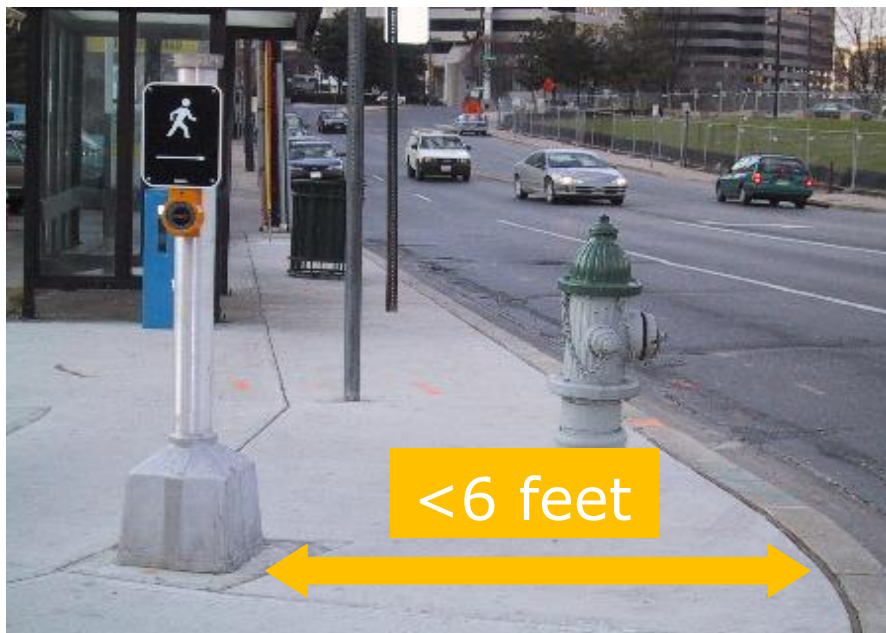
Figure 7 – Pushbutton relative to curb face
