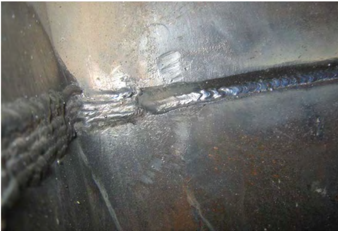
Additional passes being added to the root pass.
