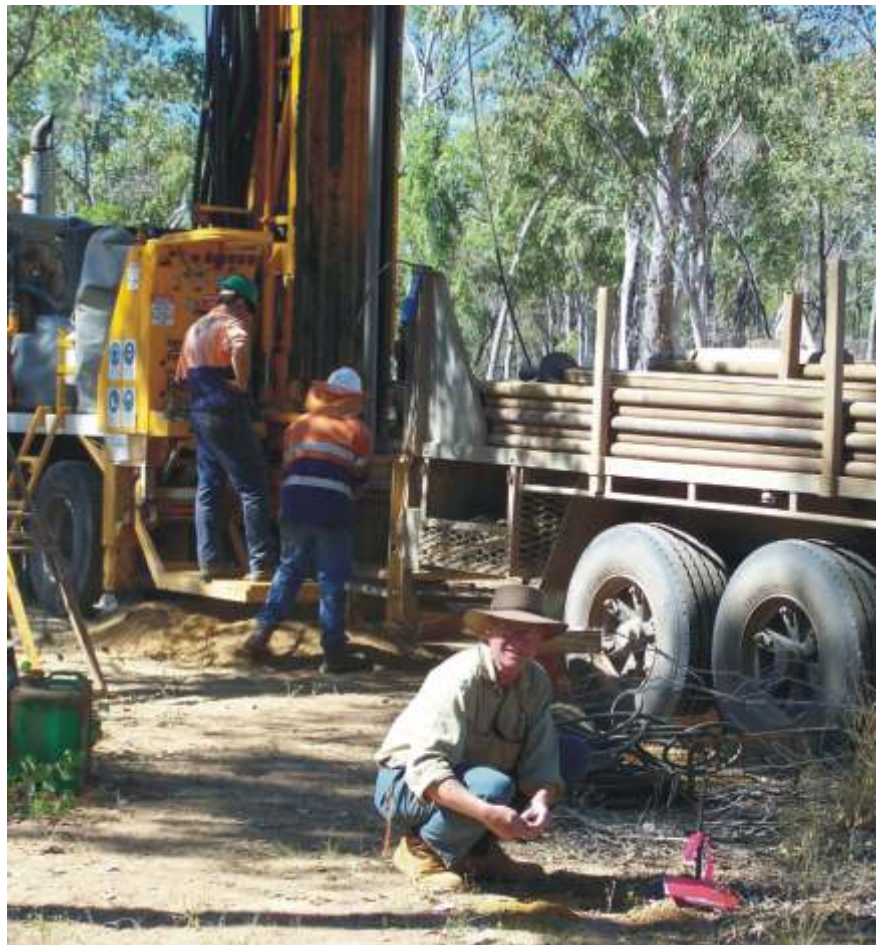
Sienna Project: drilling operations
