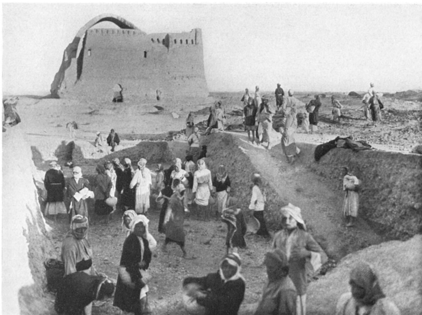
FIG. 2. WORKMEN CLEARING A TRENCH BEHIND THE PALACE AT CTESIPHON
