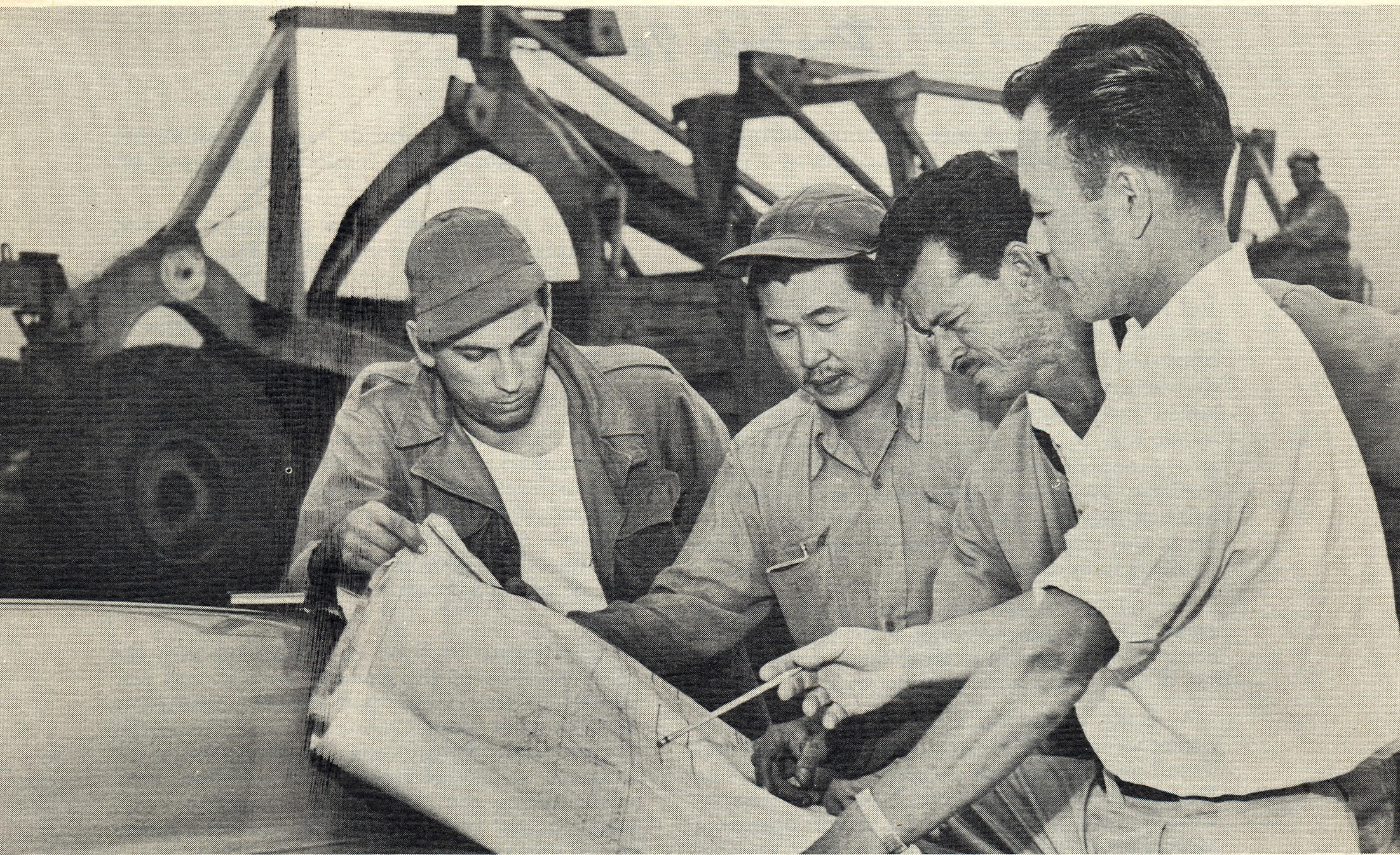
Territorial Department of Public Works Inspection Crew at Kamuela Airport Project
