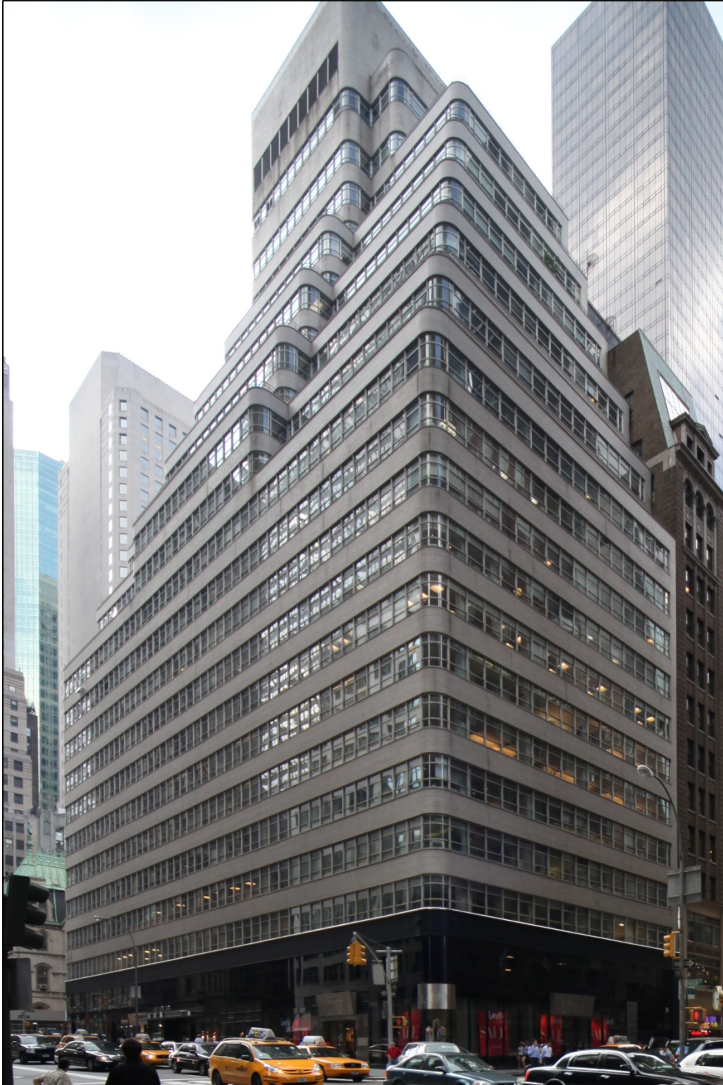
Look Building View to southwest, from Madison Avenue and 52 nd Street Photo by Christopher D. Brazee, 2010
