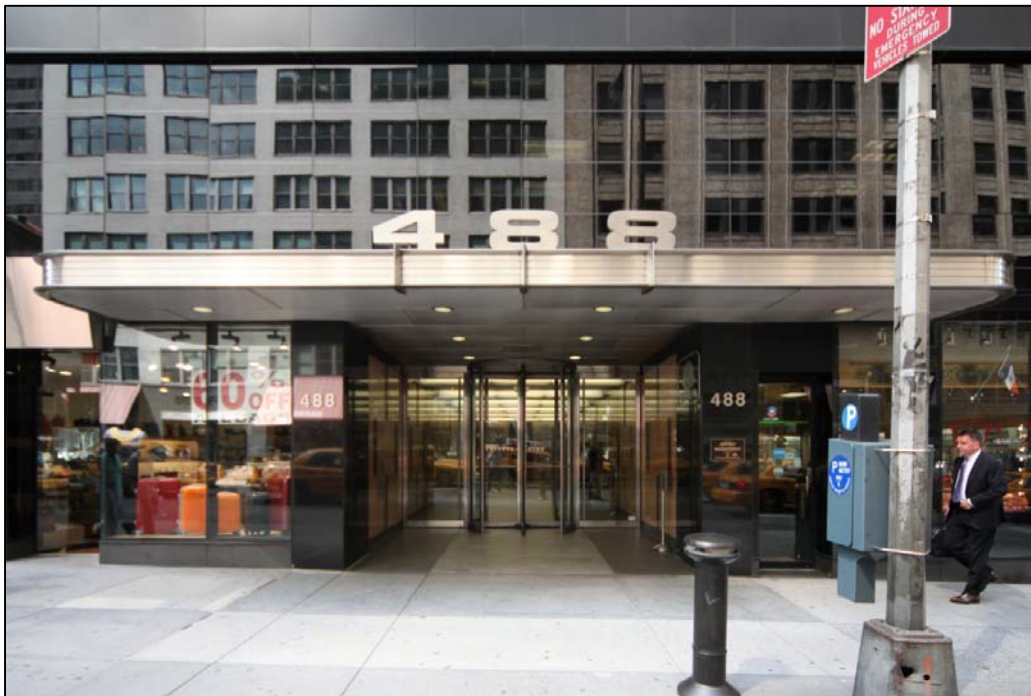
Look Building Madison Avenue facade Main Entrance Photos by Christopher D. Brazee, 2010
