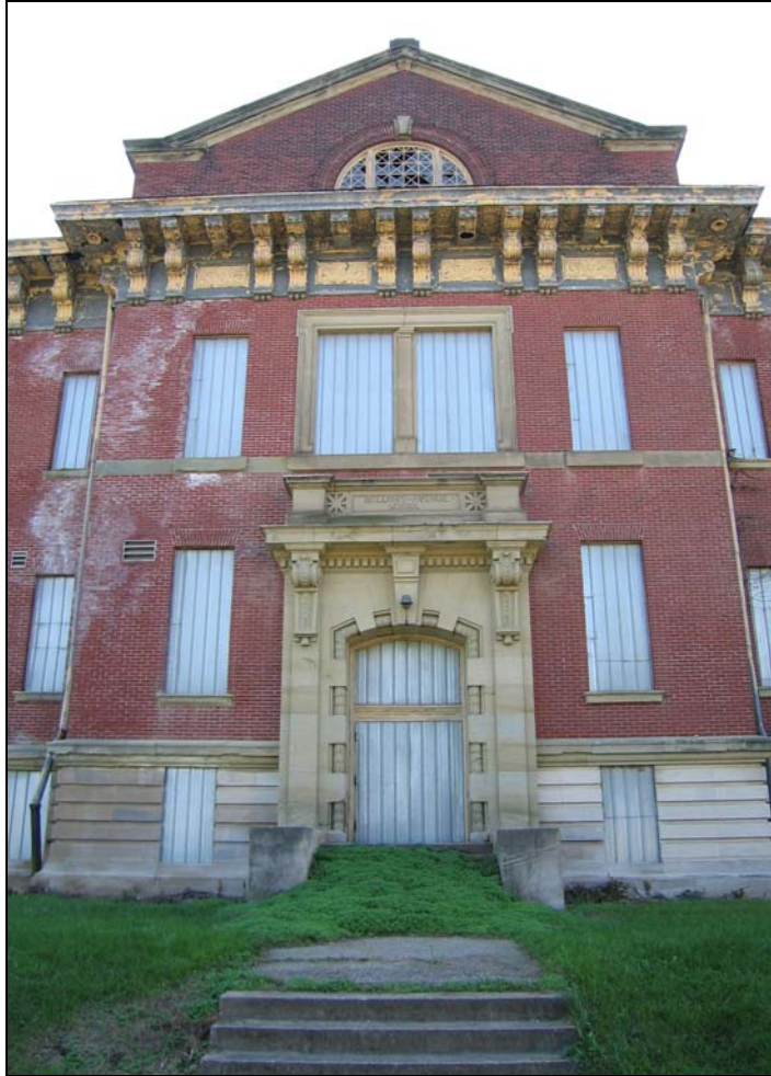
Figure 39. Bellows Avenue Elementary School, main entrance on north wall
