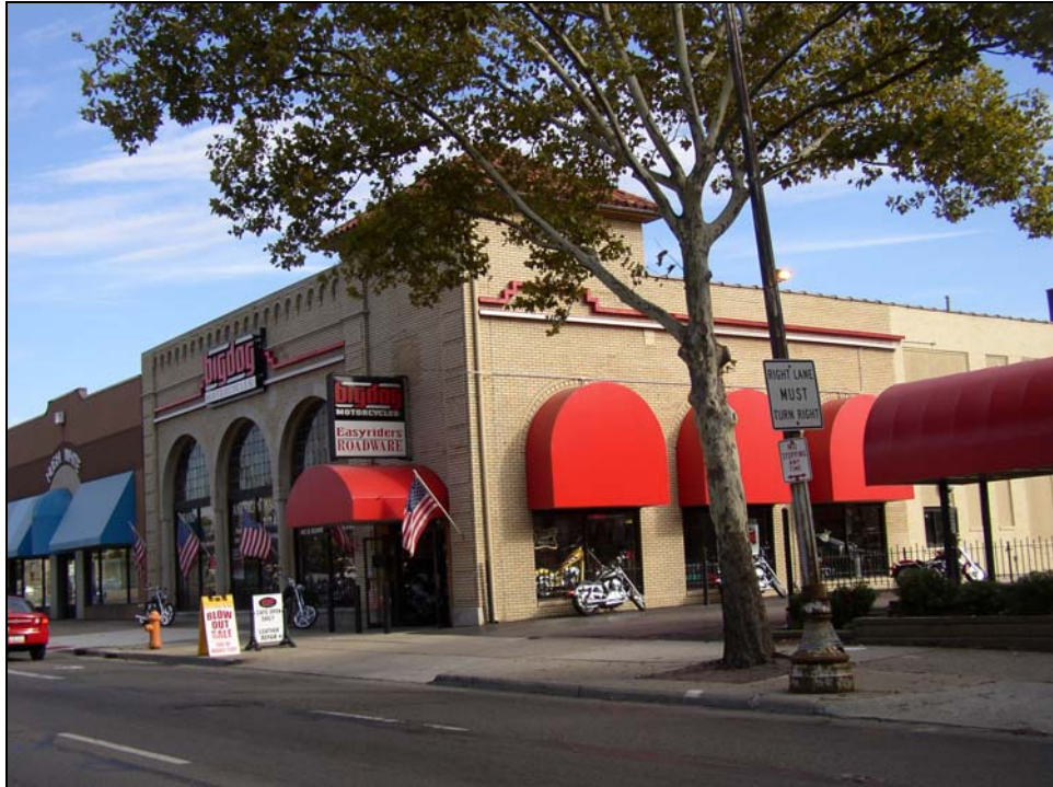
Figure 18. Former Winfield Jewell Auto Dealership at 611 East Broad Street, looking southwest
