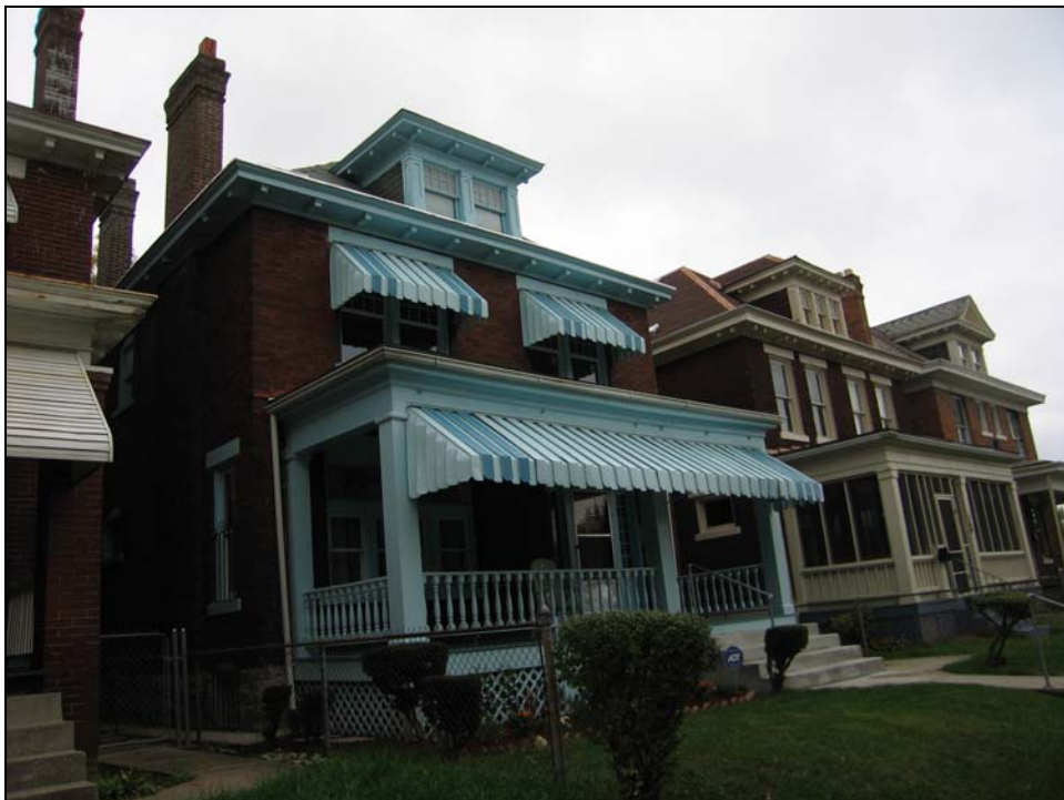
Figure 34. 540–550 Block of Wilson Avenue
