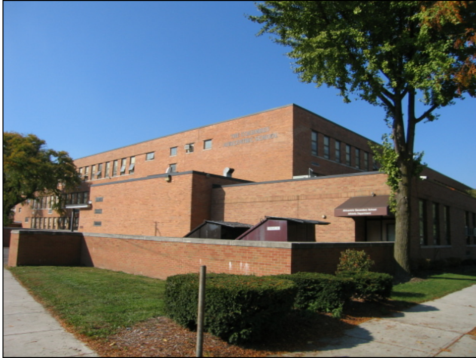
Figure 21. Mohawk School Building, looking south
