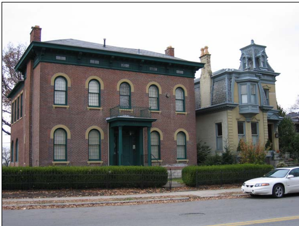
Figure 7. Partial view of East Town Street Historic District, showing 615 and 621 E. Town Street
