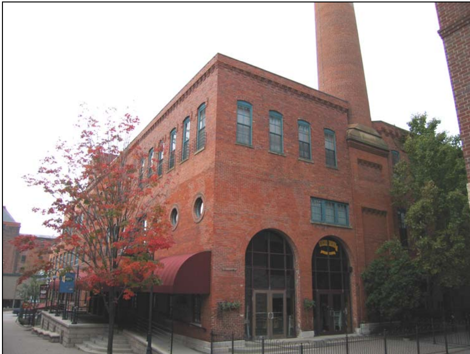
Figure 20. 444 Front Street, contributing to Brewery District (ODE)
