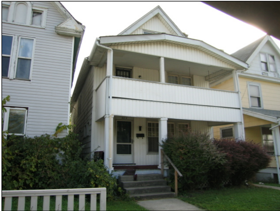
Figure 37. Area outside Old Oaks Historic District, 660 block of Miller Avenue. Note modification of houses with aluminum or vinyl siding and trim.
