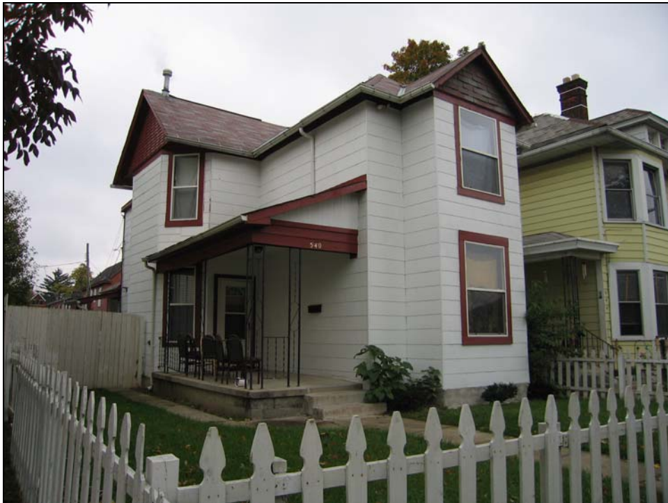
Figure 33. Champion Avenue, north of I-70. Integrity of buildings is mixed in this area, with porch, window and siding alterations very common.
