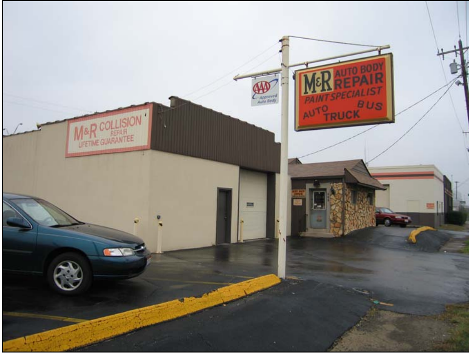
Figure 48. Block of 968 W. Mound Street
