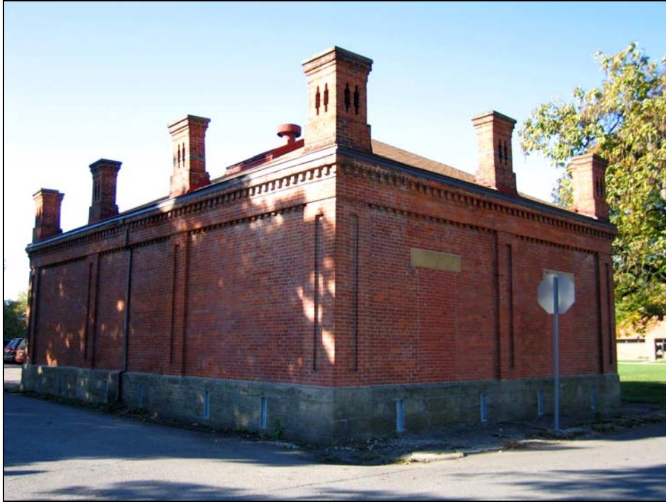
Figure 24. Building 89, the storage building/magazine at Fort Hayes
