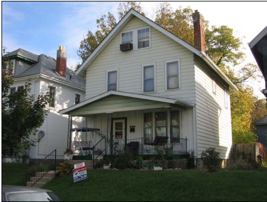
Figure 35. Kimball Place north of I-70.
