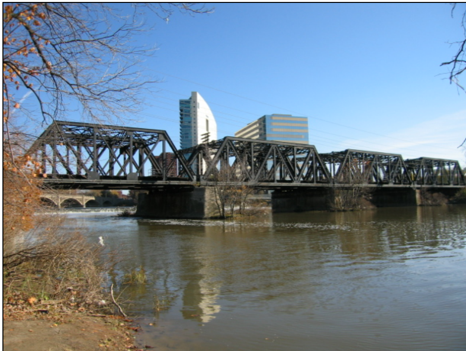
Figure 15. Scioto River Railroad Bridges, looking northeast
