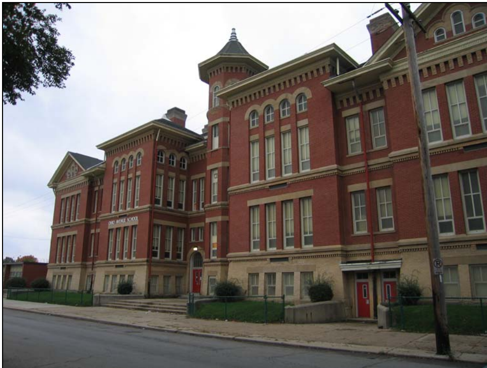
Figure 31. Ohio Avenue Elementary School, façade, looking southwest along Ohio Avenue
