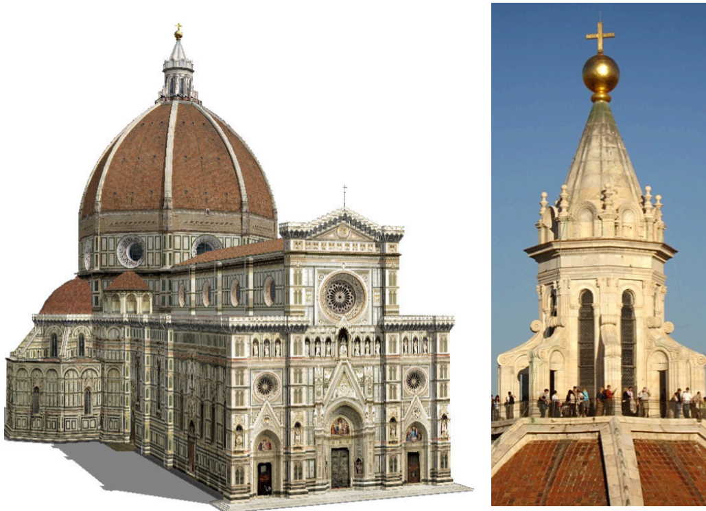
Figure 2. Left: An oblique view of the Duomo of Santa Maria de Fiore, Florence, designed by Arnolfo di Cambio in 1294, with the dome built by Brunelleschi from 1418-1436; the marble cladding was designed by Emilio de Fabris in 1871 and completed in 1887. Right: the 22 m high lantern was completed by Michelozzo in 1461, and the 8 tonne gilded copper ball was added by Verrocchio and Leonardo da Vinci in 1469.
