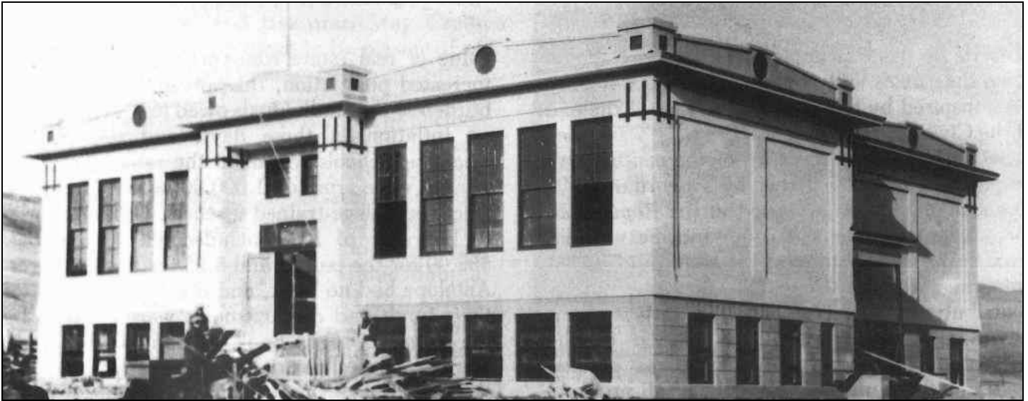
Figure 6: Antelope School, nearing completion, likely taken in fall, 1924 50
