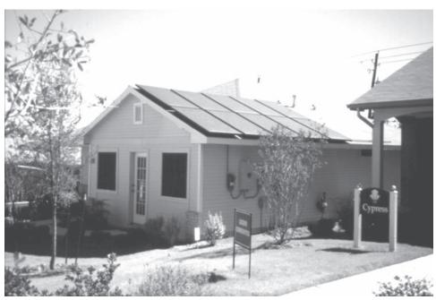
**RESIDENTIAL PV SYSTEM** The solar panels on the roof produce electricity that travels through wires to the distribution panel on the side of the home.
