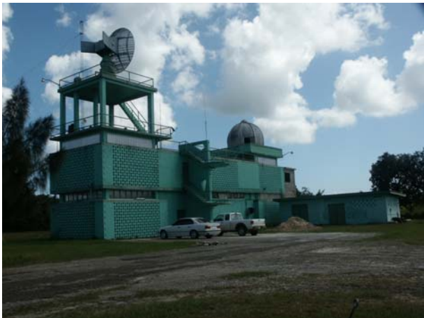
Fig. 53: National Meteorological Service The NMS building at the Belize City airport
