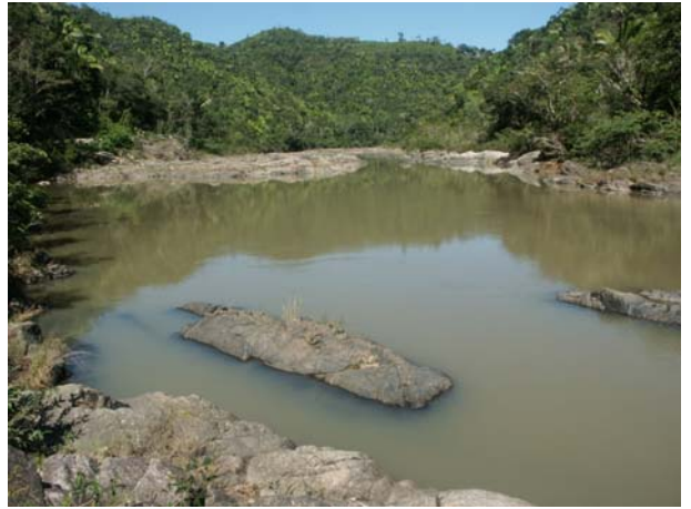
Fig. 16: Vaca Falls Dam Site - Downstream The picture shows the river bed downstream of the dam axis with another Vaca Falls rock sill. Downstream of this sill would be located the powerhouse of the diversion alternative.
