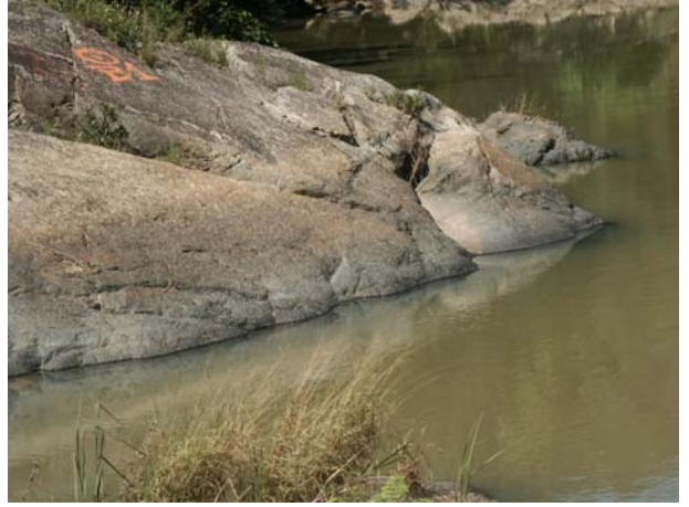
Fig. 14: Vaca Falls Dam Axis - Left Abutment Impoundment alternative. Left abutment with the dam axis benchmark B1. The outcropping massive granite shows favorable conditions for dam foundations.
