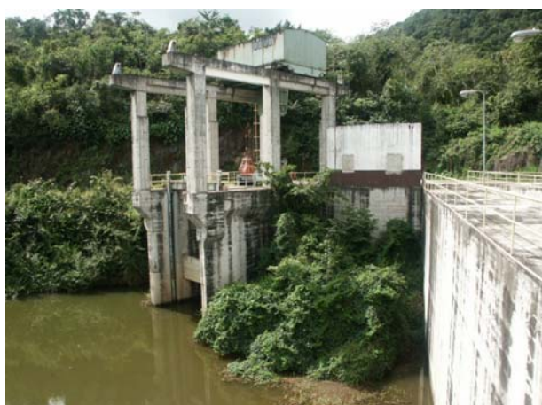
Fig. 9: Mollejon Low Pressure Tunnel Intake
