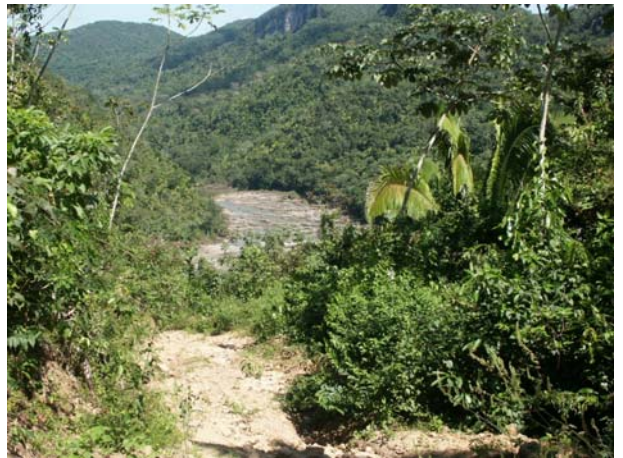
Fig. 18: Vaca Falls Powerhouse Site A few hundred metres downstream of the contemplated dam axis, the powerhouse site of the diversion alternative. Less favorable morphology for a 10 m higher dam.
