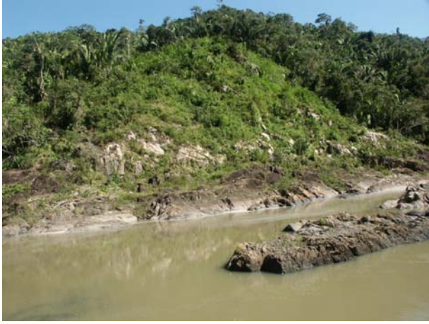
Fig. 13: Vaca Falls Dam Site on the Macal River Impoundment alternative. Gravity dam: Normal water level at EL 143.5; Crest at EL 150; Toe at EL 90. right abutment area where the forest has been felled. Rock sill of the so-called Vaca Falls.
