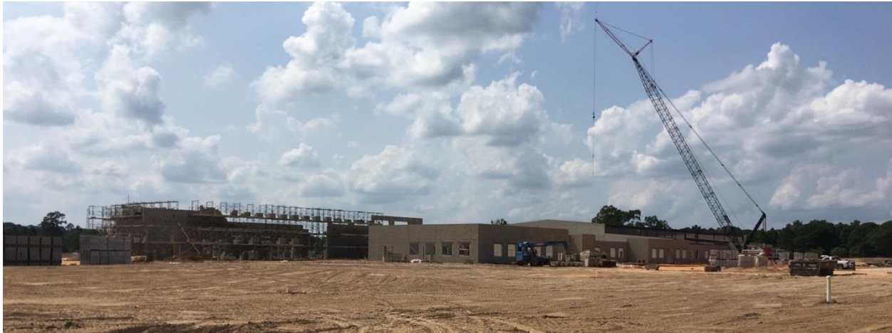
Construction Underway at MISD's Newest Elementary.....Keenan Elementary
