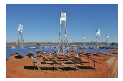
Each of the SSR's are effectively an on demand steam generator, which is connected by a steam manifold that delivers the steam to the balance of plant and a  $3MW_e$  steam turbine generator, which is in turn connected to the Australian National Electricity Market.
