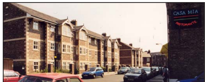
• Middleton Court, Hutton Terrace
