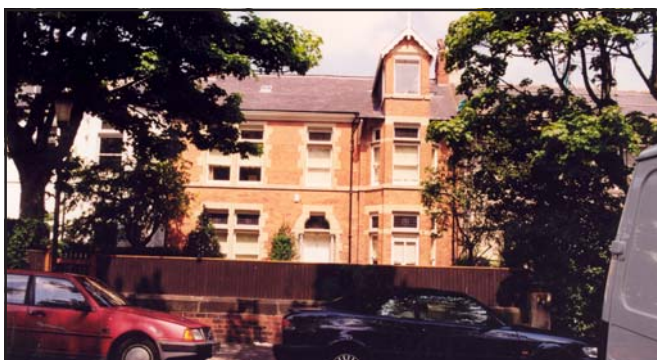
● Red brick houses on Osborne Avenue
