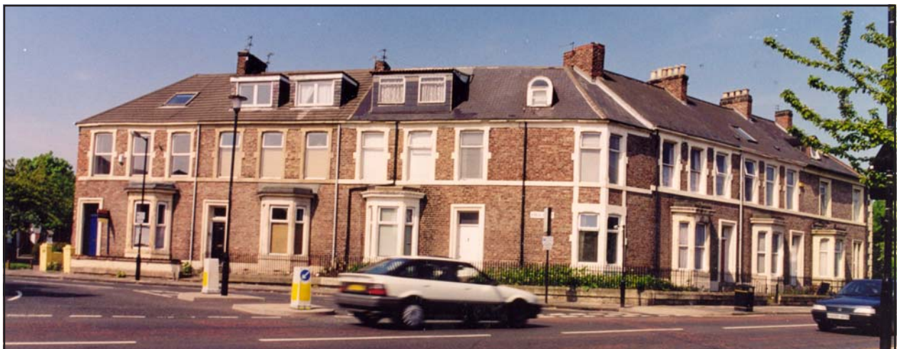
● Shield Street/Portland Road
