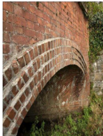
Bandon Skew Bridge
