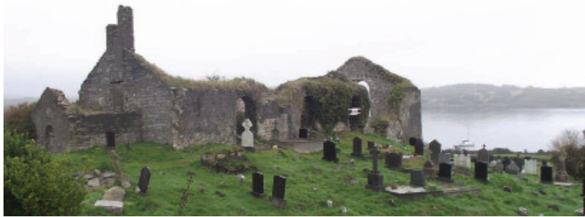
Schull Church and Walkway
