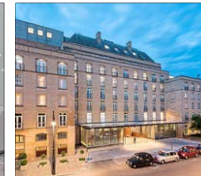
Forward-looking design: the elegant addition, with specially crafted glass and cantilevers, spans the frontage's full width
