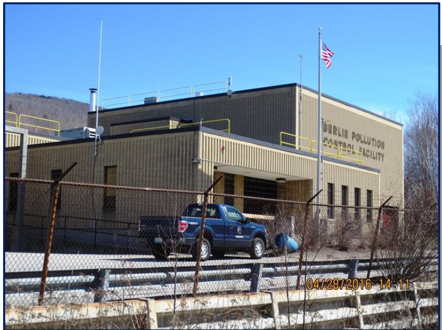
The Berlin Waste Water Treatment Plant. Photo Credit: New Hampshire.
