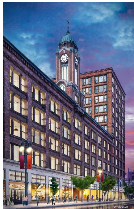
The Sibley Building. Image Credit: NYSERDA.
