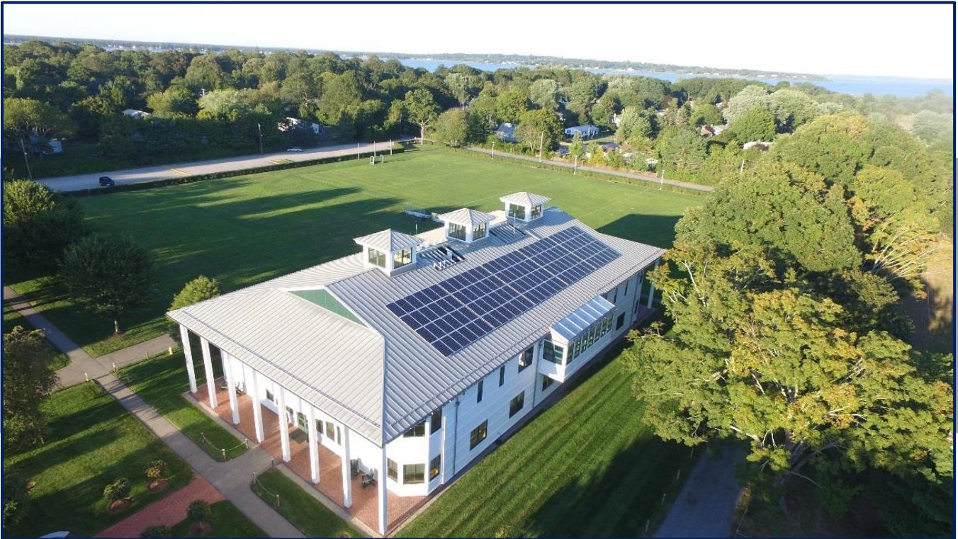
Rocky Hill School with rooftop solar array. Photo credit: Peter Frost, Rocky Hill School parent.
