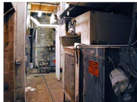
Typical aging infrastructure (Quinn Building)
