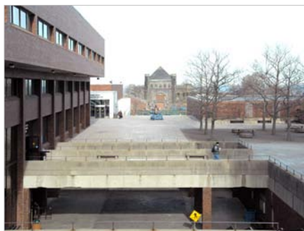
Existing obstructed path to Calf Pasture Pumping Station
