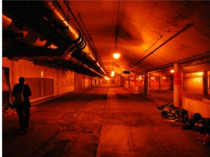
View of existing Substructure interior
