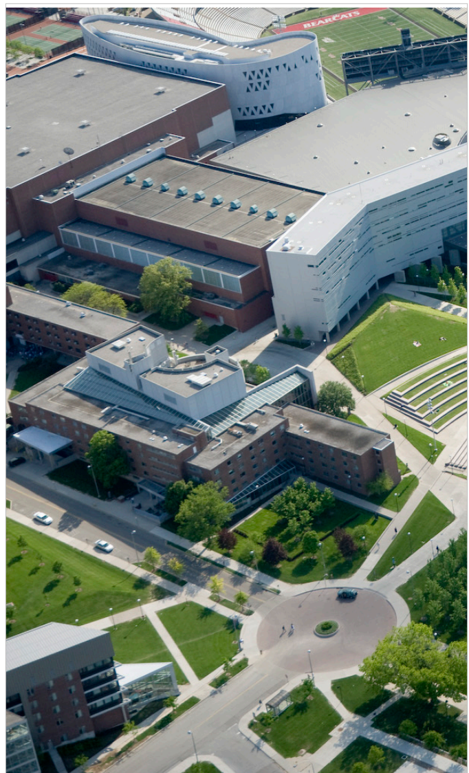
Accessible campus quad between buildings and grade changes, University of Cincinnati
