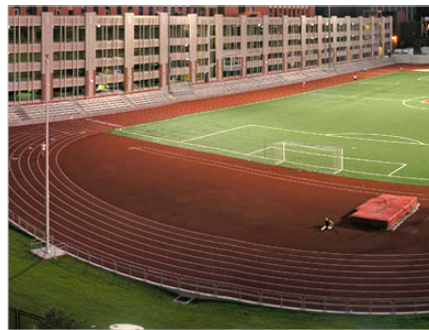
Garage & bleachers facing track & soccer field, Univ. Cincinnati
