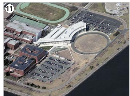
Current main entrance at Campus Center (Source: maps.live.com )
