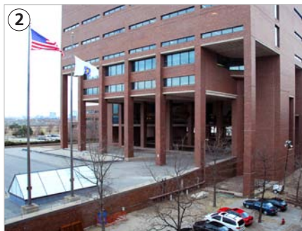
2 Healey Plaza, the roof of the Utility Plant, sliding under Healey
