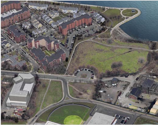
Existing intersection of Mt. Vernon Street and campus loop road
