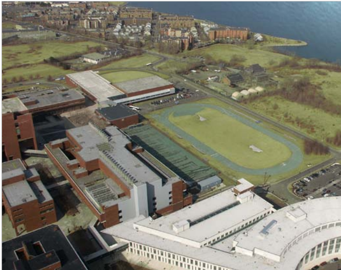
Campus tennis courts (currently used as a parking lot) and the running track/soccer field
