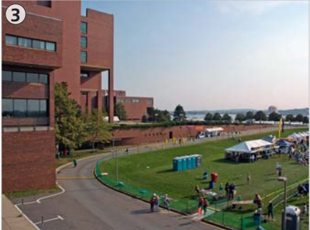
Vehicular ramp over Utility Plant to plaza above Substructure
