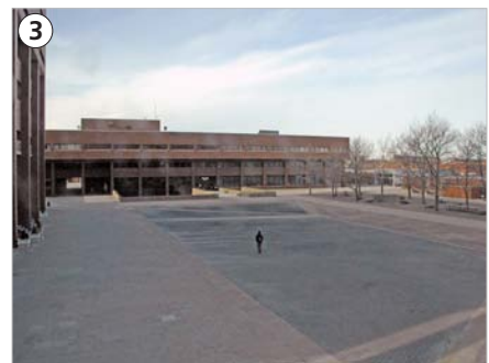
3 Existing central plaza, the roof of the Substructure
