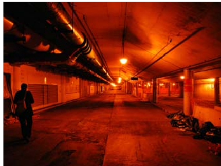
View of existing Substructure interior
