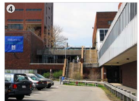
Stair to and over Substructure and to Central Plaza
