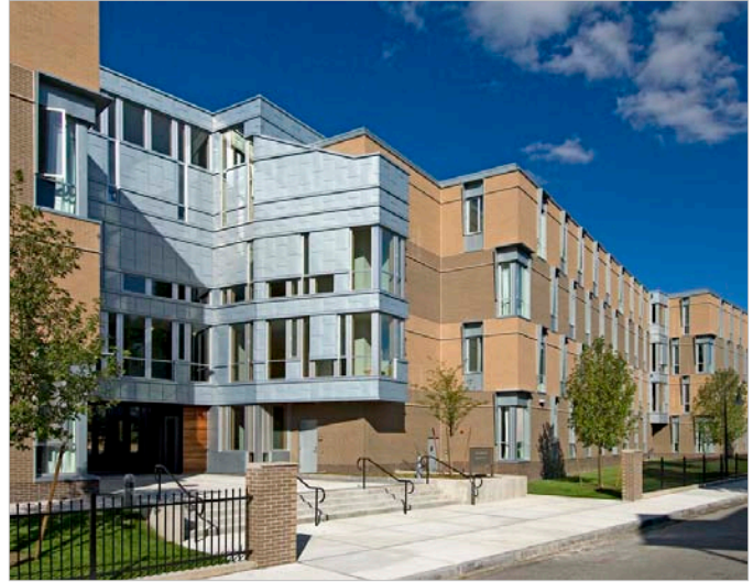
Student residence hall flanking campus portal facing city street, Clark University
