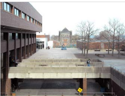
On-grade, through-campus path after Substructure is demolished
