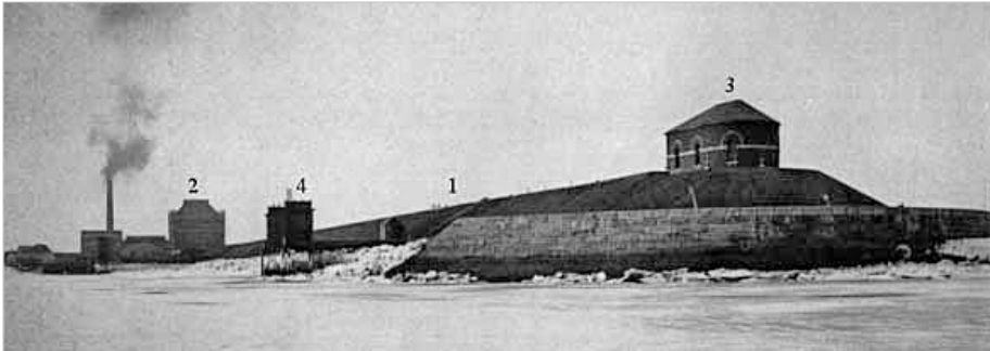
Entrance pavilion (3) to the covered outfall tunnel (1) leading from the Pumping Station (2) (Source: Gaining Ground by N. Seasholes)
