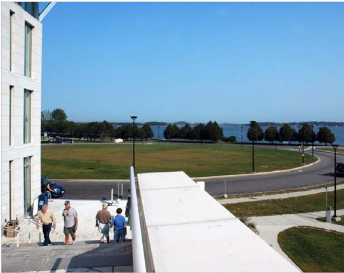
Existing view towards East Harbor Common beyond the Campus Center driveway oval
