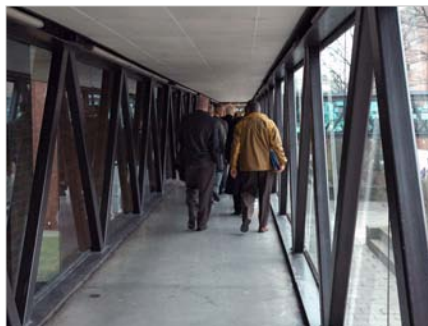
Existing catwalk interior along Science Center
