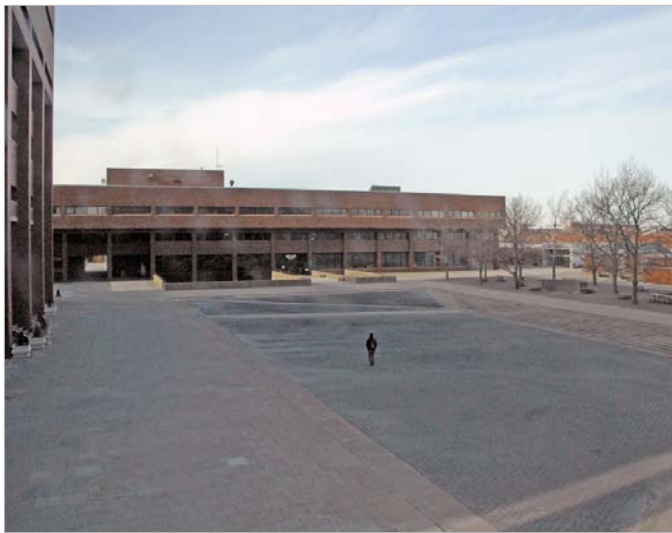
Existing elevated campus plaza on the roof of the substructure
