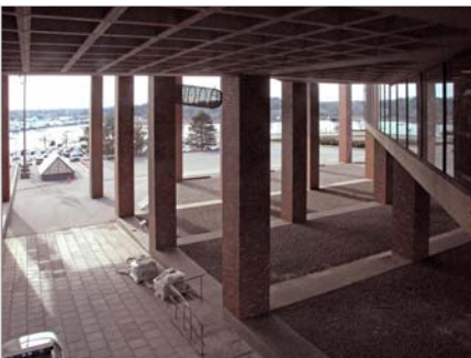
Void under Healey Library that may be infilled for new space
