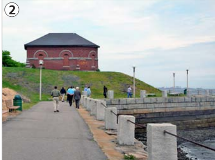
Access building to outfall tunnel at east edge of HarborWalk
