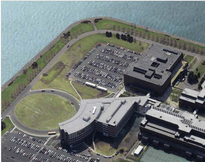
Site S today with the Campus Center and Science Center in the foreground
