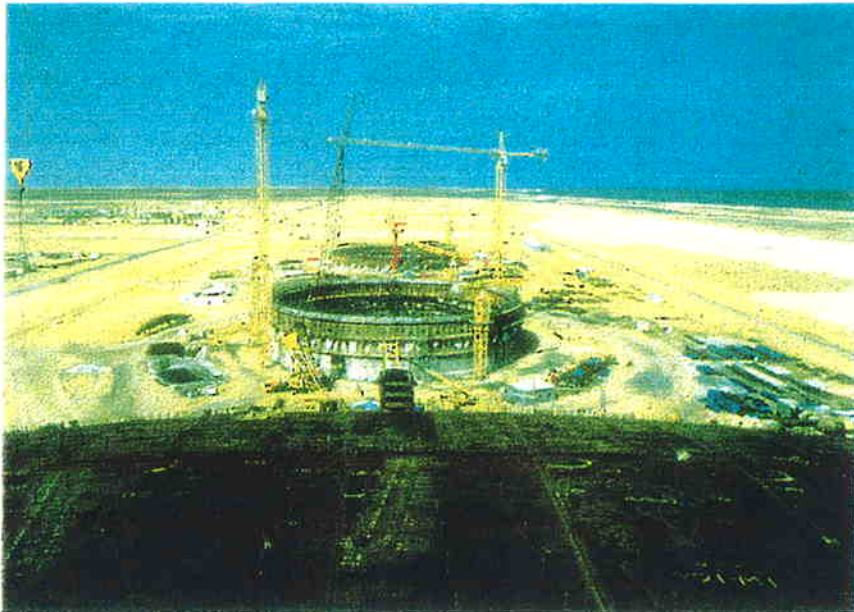
▼ Tanks 2 and 3 under construction
