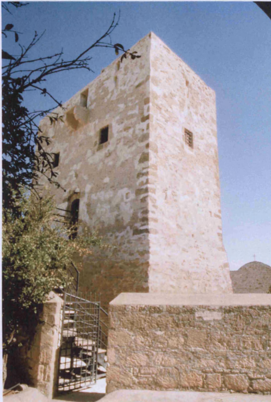
West face with entry at first floor level.
