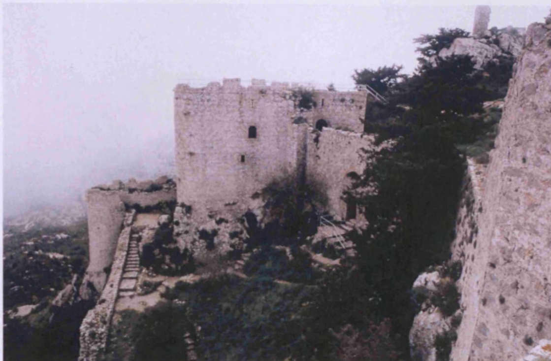
South end of the east front. The large D-shaped tower (2 on plan) has a lesser outwork beneath it. This is a narrow horse-shoe shaped fighting platform (32 on plan).
