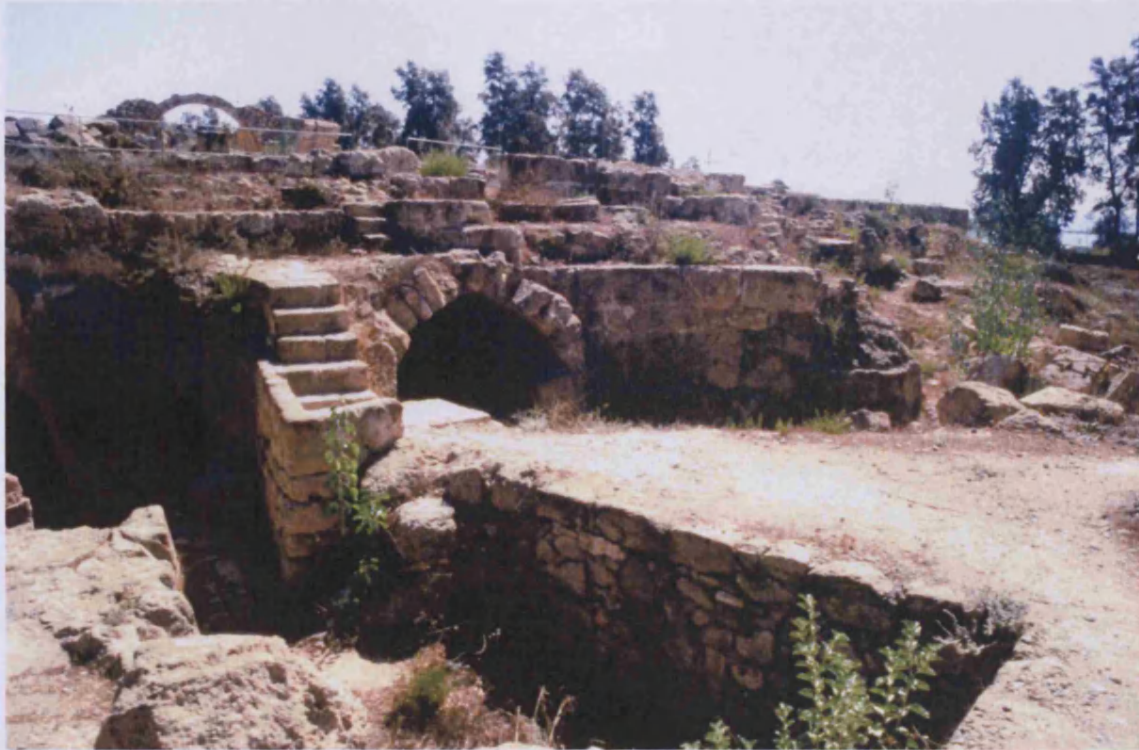
Cut-water tower (C on plan) and postern, as altered, on west outer enceinte .
