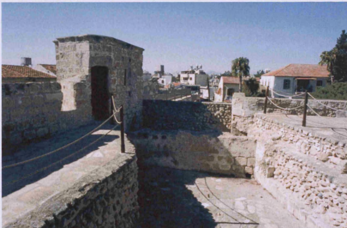
South end of the pentagonal work and adjoining wall (1 on plan). The raised walkway and sentinel turret on the south (left on the photograph) is later – Venetian/Ottoman work.
