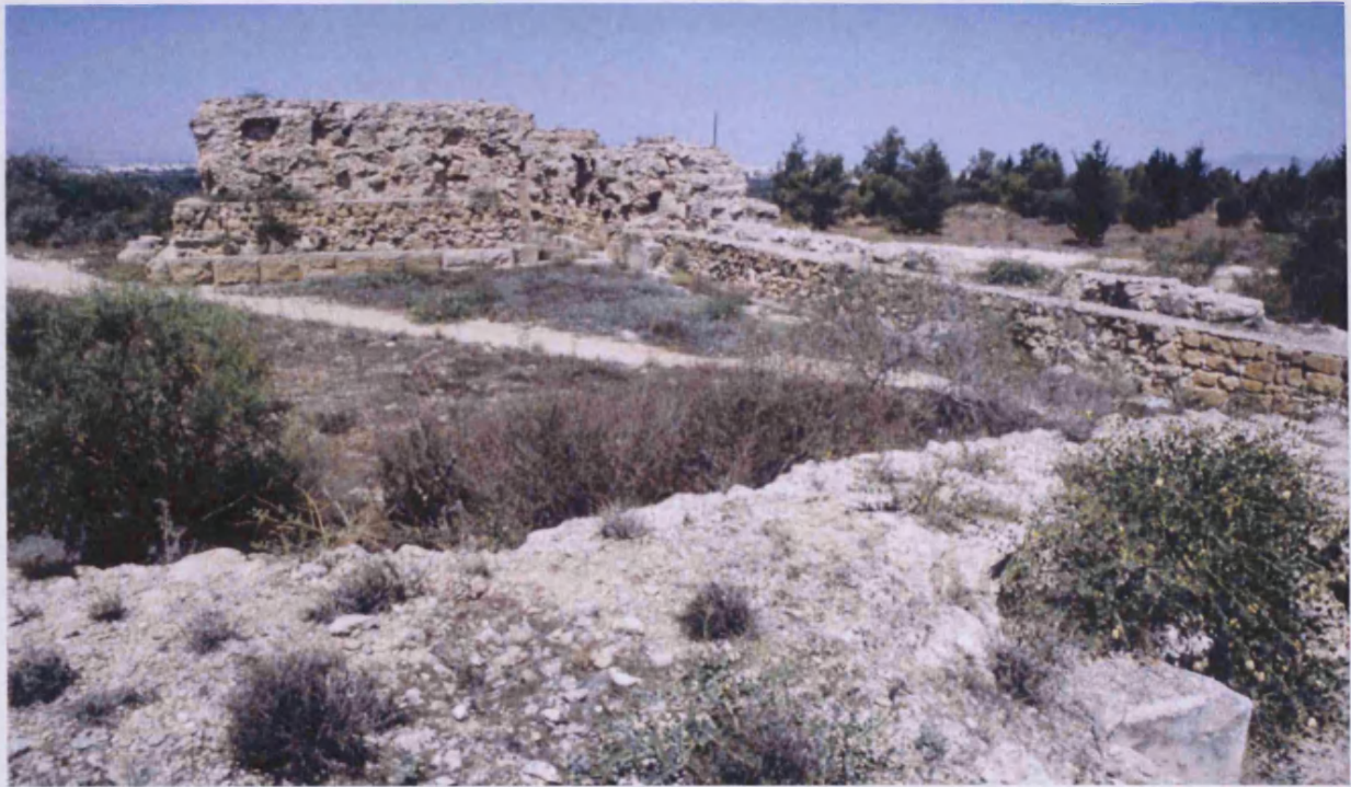
West tower and the central wall connecting to the east tower.
