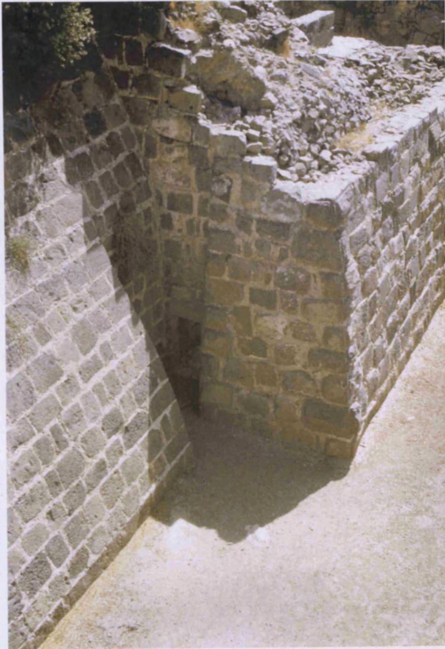
Belvoir. Note the substantial batter of the outer enceinte providing for concealment of sally ports.
