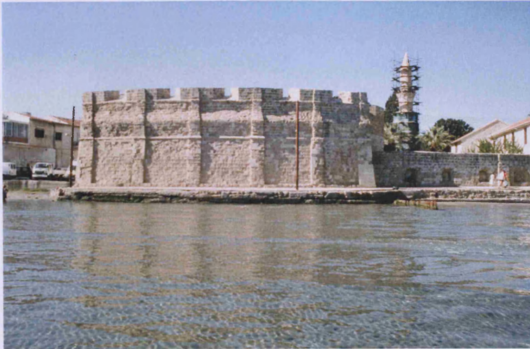
East (seaward) wall showing main Venetian and Ottoman artillery block incorporating and masking the medieval pentagonal work on this side (2 on plan).
