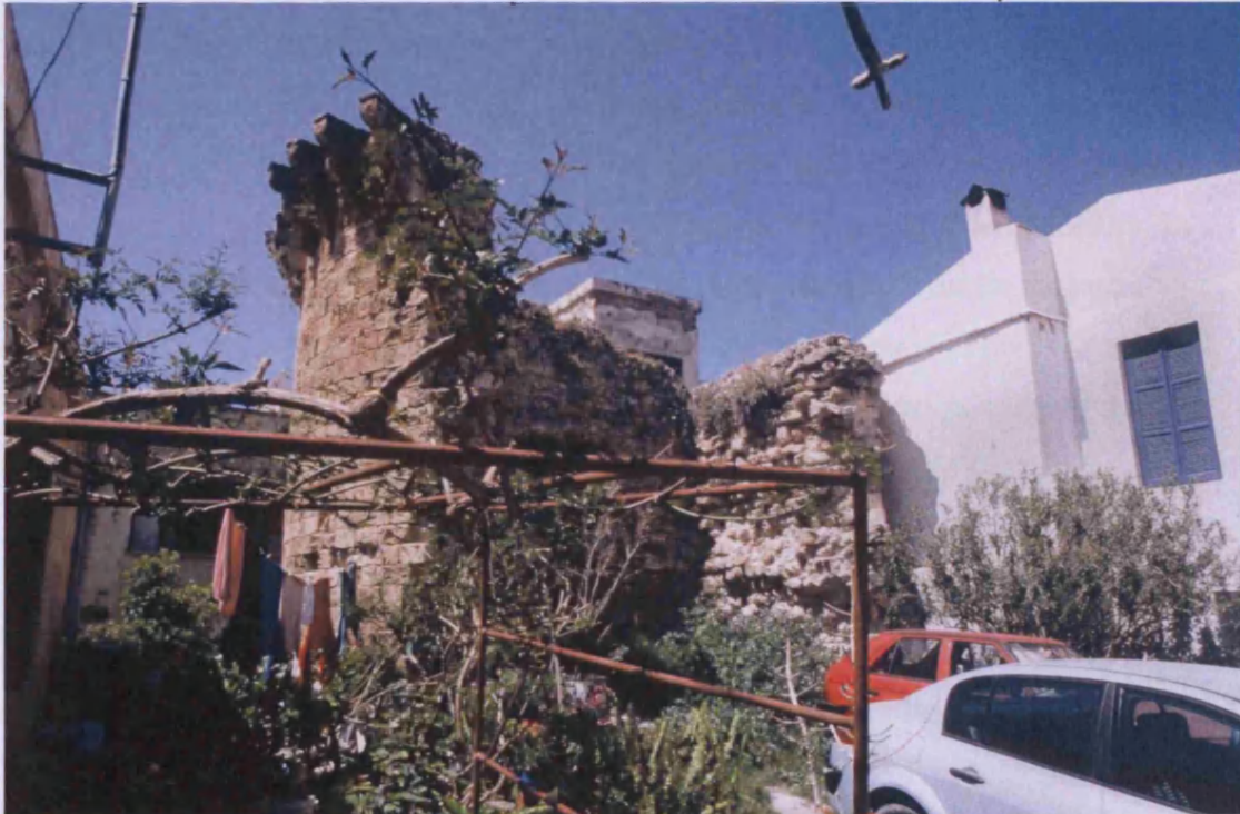
D-shaped tower (B on plan) on the town's west wall, possibly one of a pair protecting an entrance between. The elaborate corbels for machicolation are apparent, suggesting a late fourteenth or fifteenth-century date for this elaboration.
