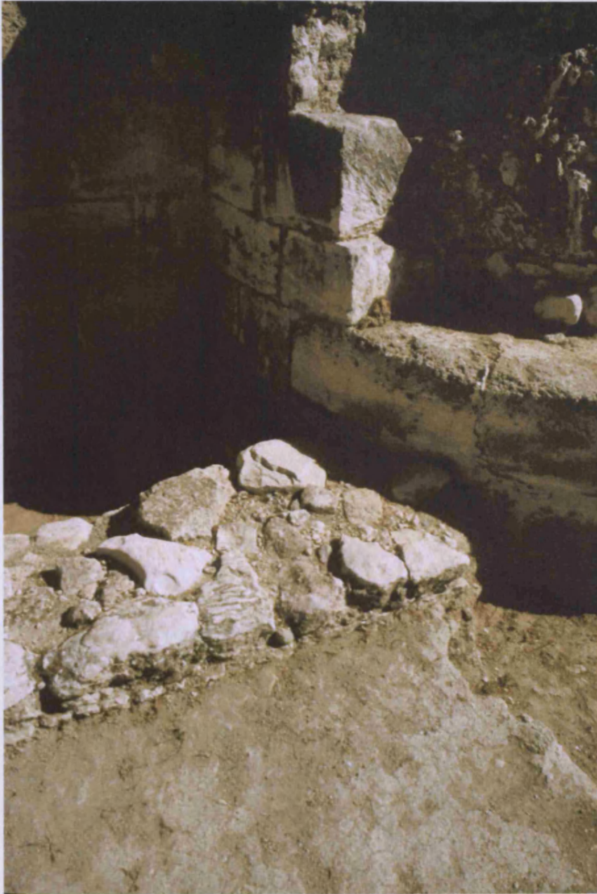
Detail of the junction of the outer, early wall (1 on plan) with the fifteenth-century cylindrical tower (2 on plan) on its north side. They are clearly not articulated and built at different times, the tower being of a piece with the later, thicker wall lying behind (3 on plan).
