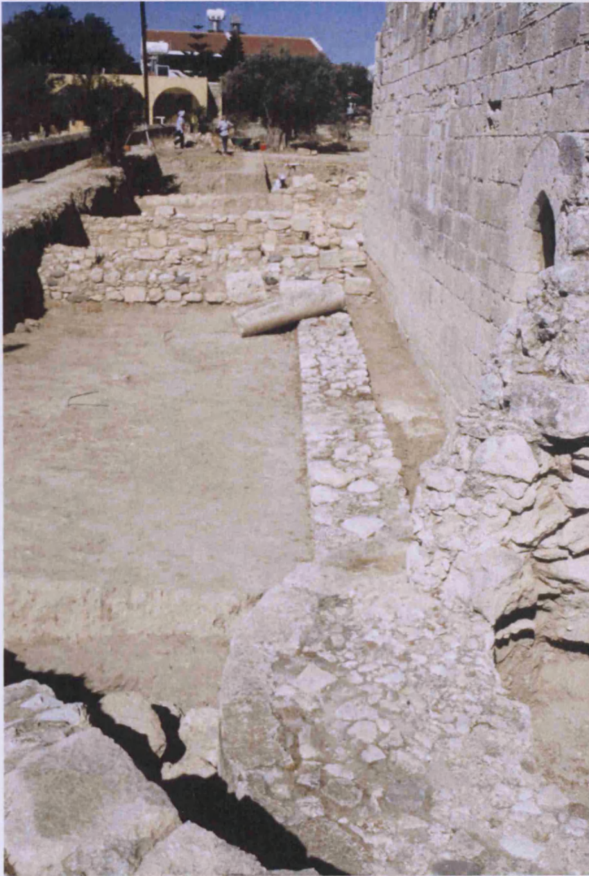
View of earlier 'castle' wall (1 on plan) as now excavated, lying beyond the west wall (3 on plan) of the fifteenth-century compound.
