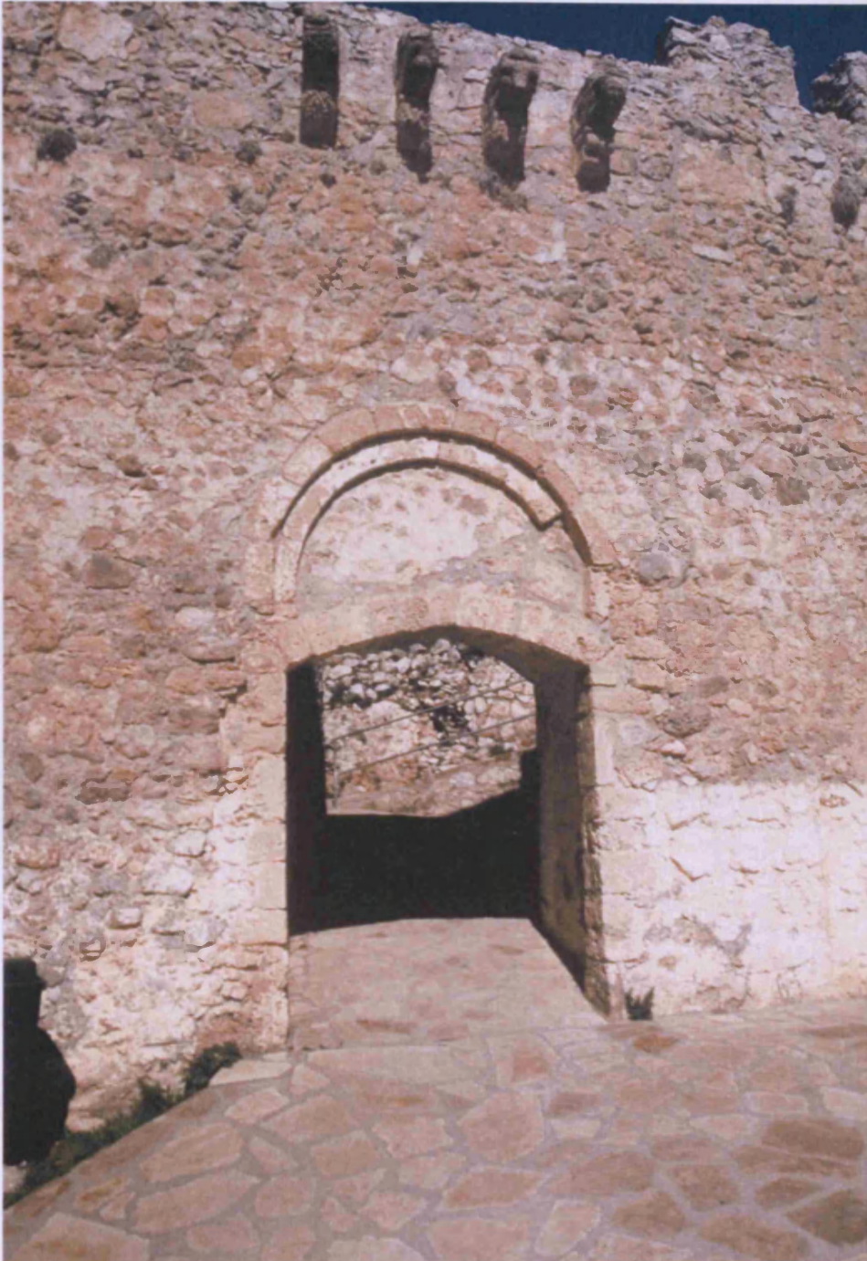
Entrance (5 on plan) through main lower ward curtain, showing Byzantine arch over later arch, with corbels above for a box machicolation.
