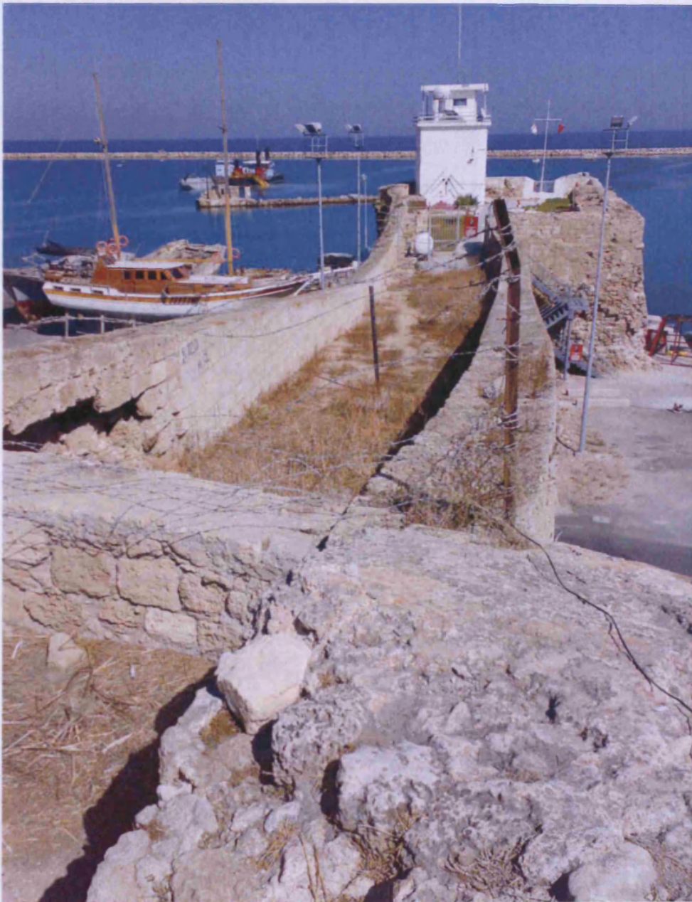
Venetian fortified corridor-breakwater from castle to port tower.
