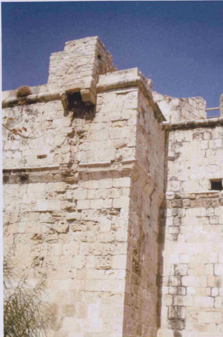
Latrine brattice at roof level on the post medieval outer casing on the fort's south-west side.
