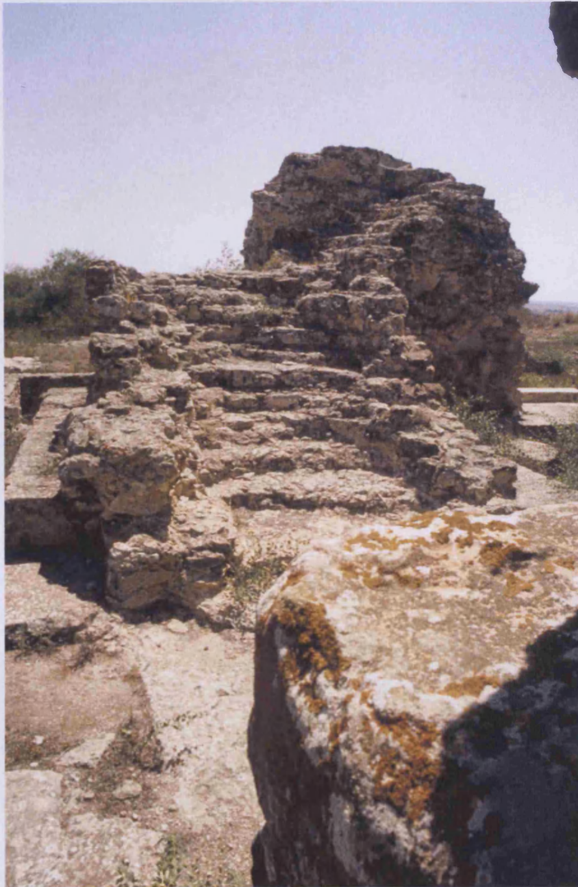
Steps in north-east angle of west tower.
