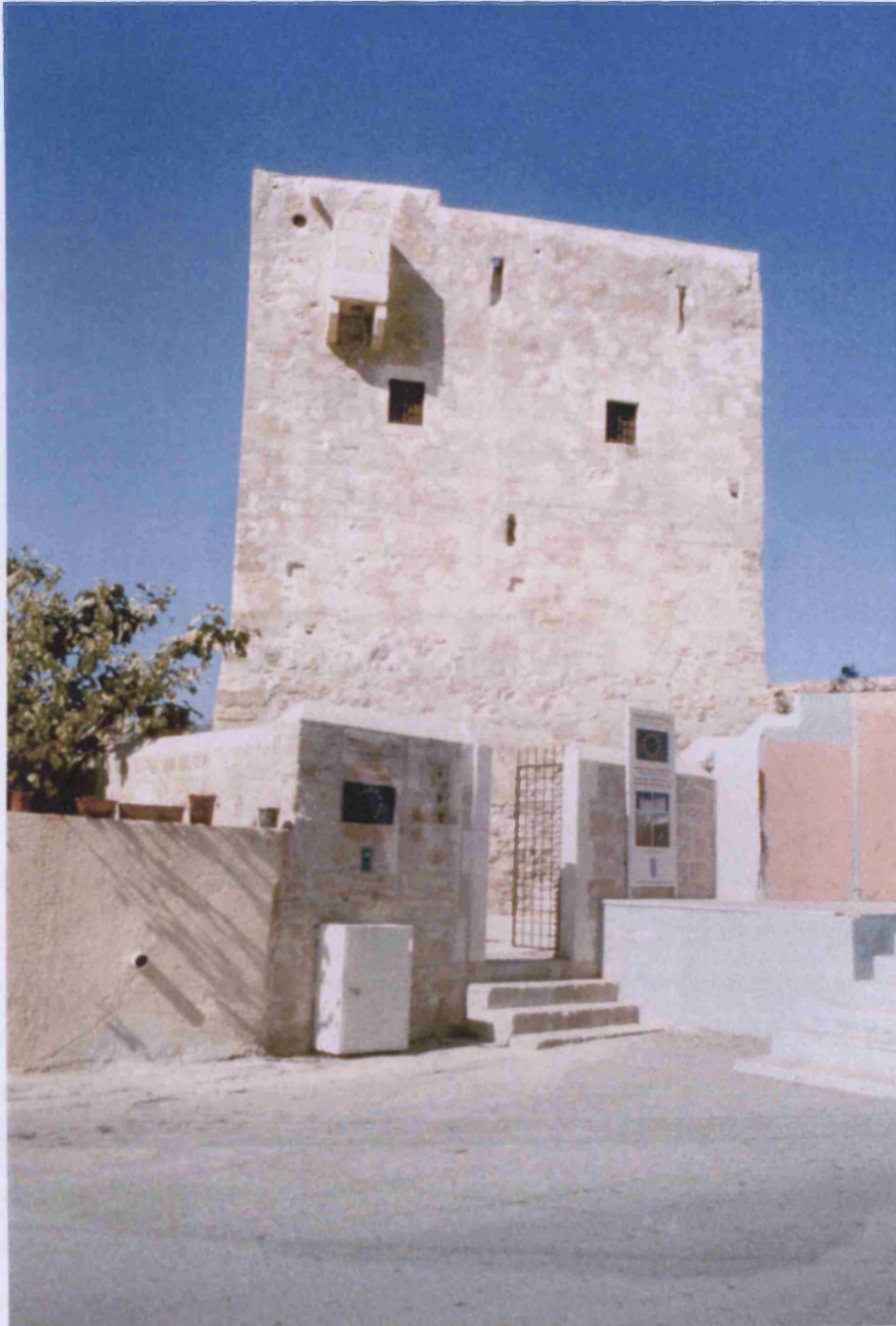
East face with latrine at roof level.
