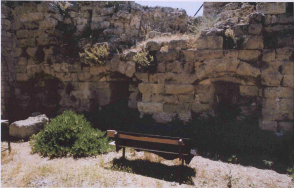
Interior of west curtain – south section: archères on two levels.
