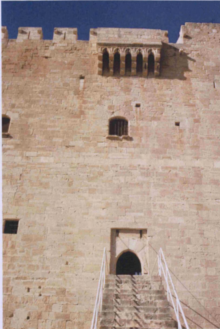
Close up of south (entry) face of fifteenth-century keep showing first floor entry and ornate box machicolation.
