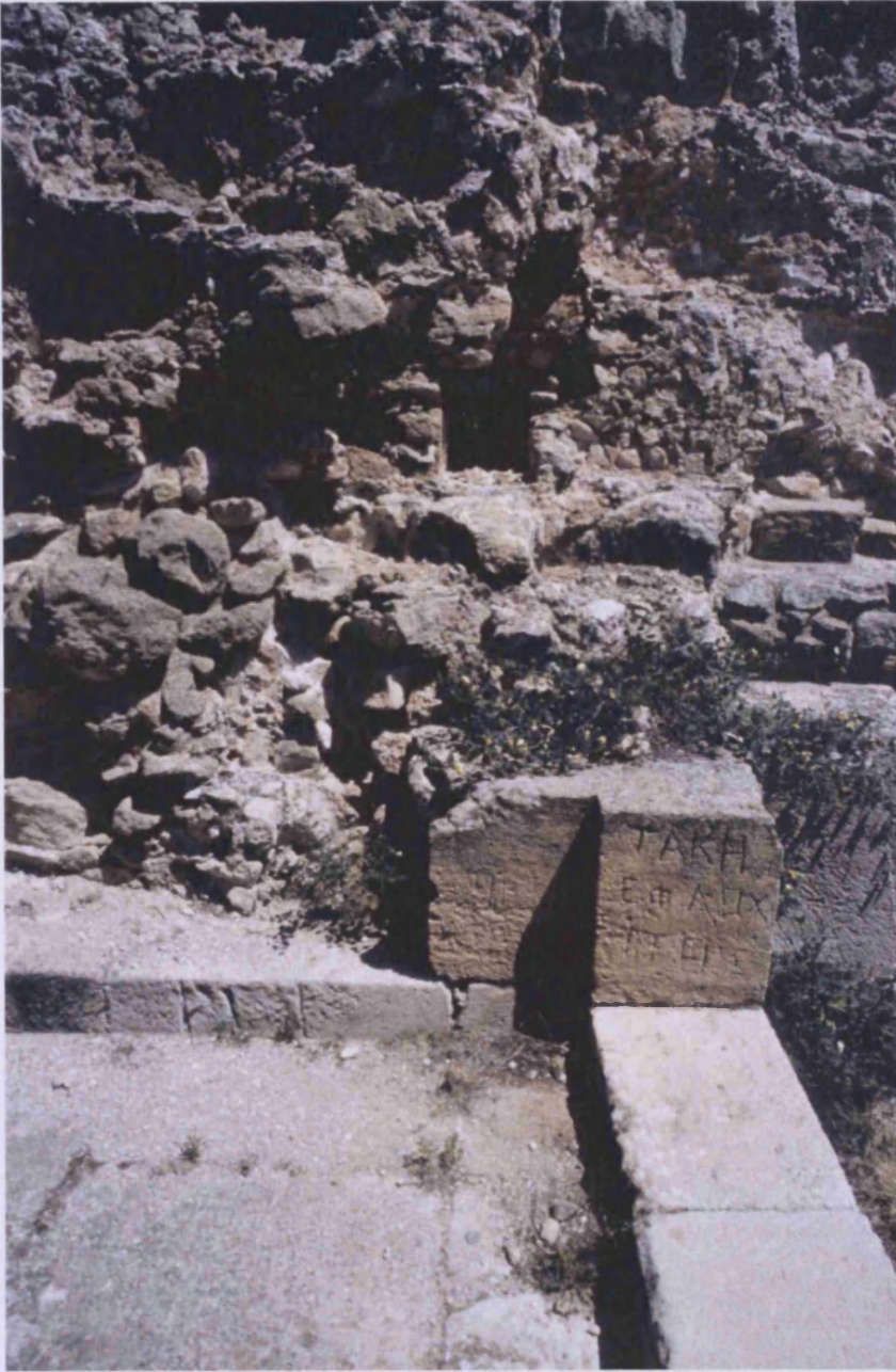
Main entrance to west tower, showing drawbar slot and remains of rebate for door. This photograph was taken in June 2007 – compare with La Cava 3 above from October 2006.
