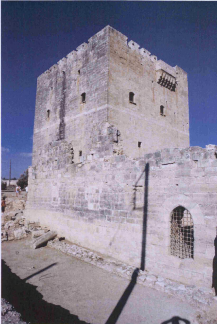
General view of the keep and compound wall of the early 1450s from the south-west. The earlier wall (1 on plan) located outside the fifteenth-century compound wall on the west can be seen in the foreground. Columns, most likely brought to the site to serve as a means of strengthening these earlier walls, may also be noted.
