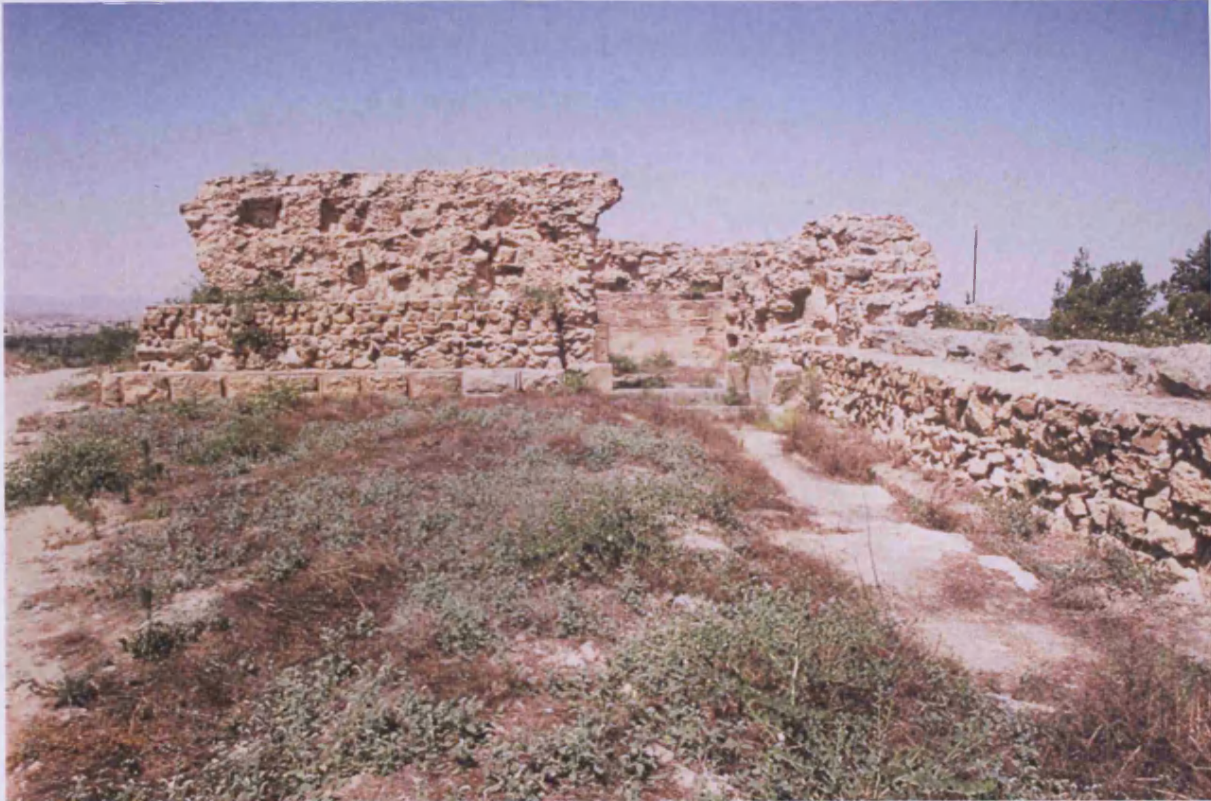
West tower and central wall, showing main entrance to the tower on its east side.
