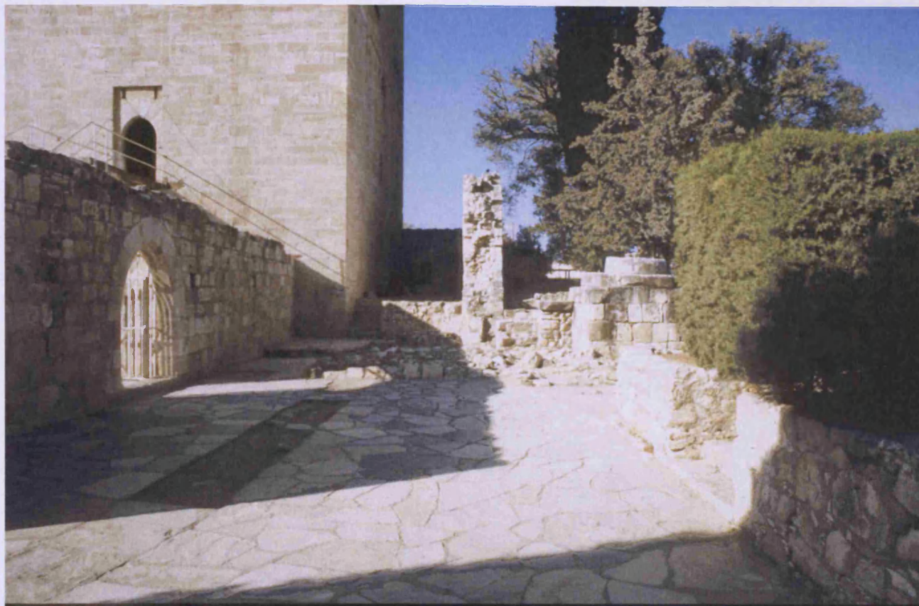
Profile of fifteenth-century wall (10 on plan) on the east side of the keep at its junction with the earlier apsidal tower (5 on plan) containing a well. In the foreground, the base of an early, less substantial wall (4 on plan) can be traced following a line a little to the west. Within that (on the left of the photograph) the present compound wall dates from the restorations of the 1930s.
