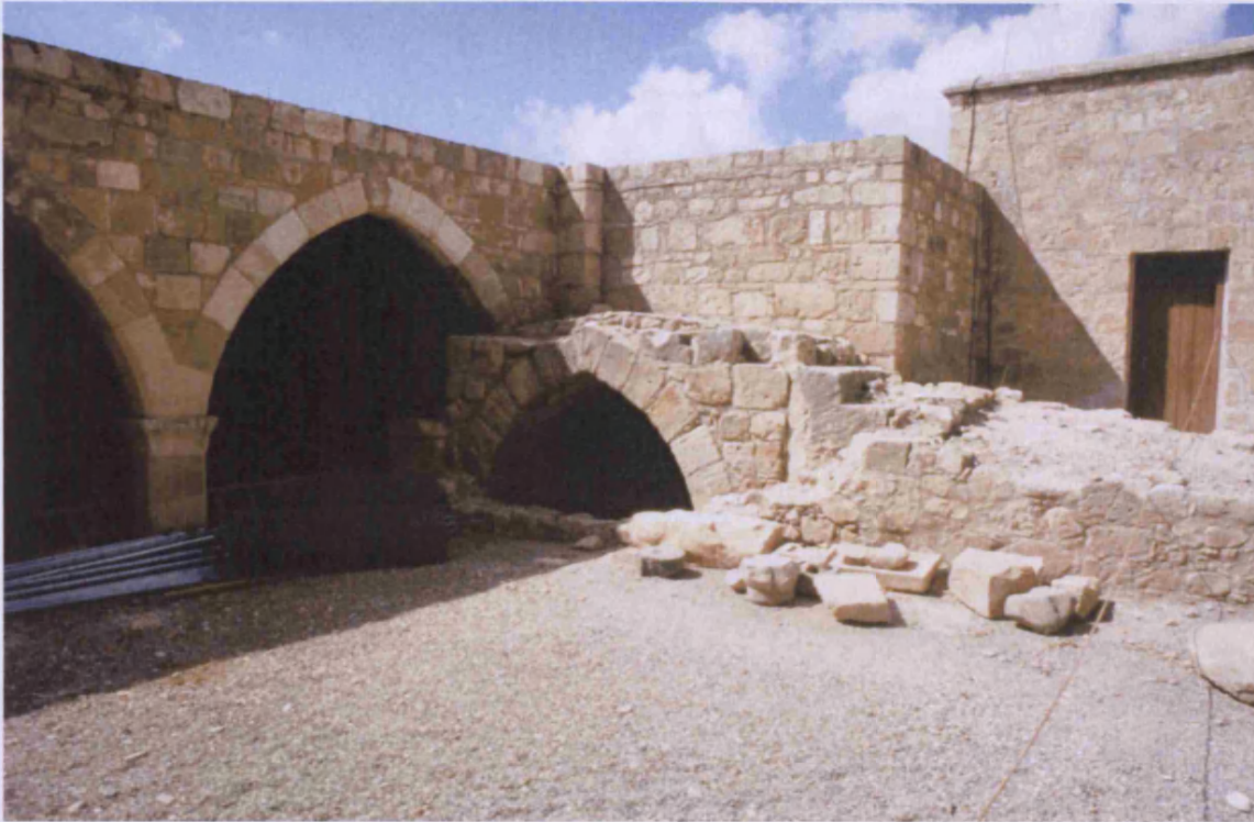
South-west corner of courtyard. On the east side, an arch supported a ramp (4 on plan) leading to the upper storey. The westernmost arch of the restored south range can be seen at a higher level.
