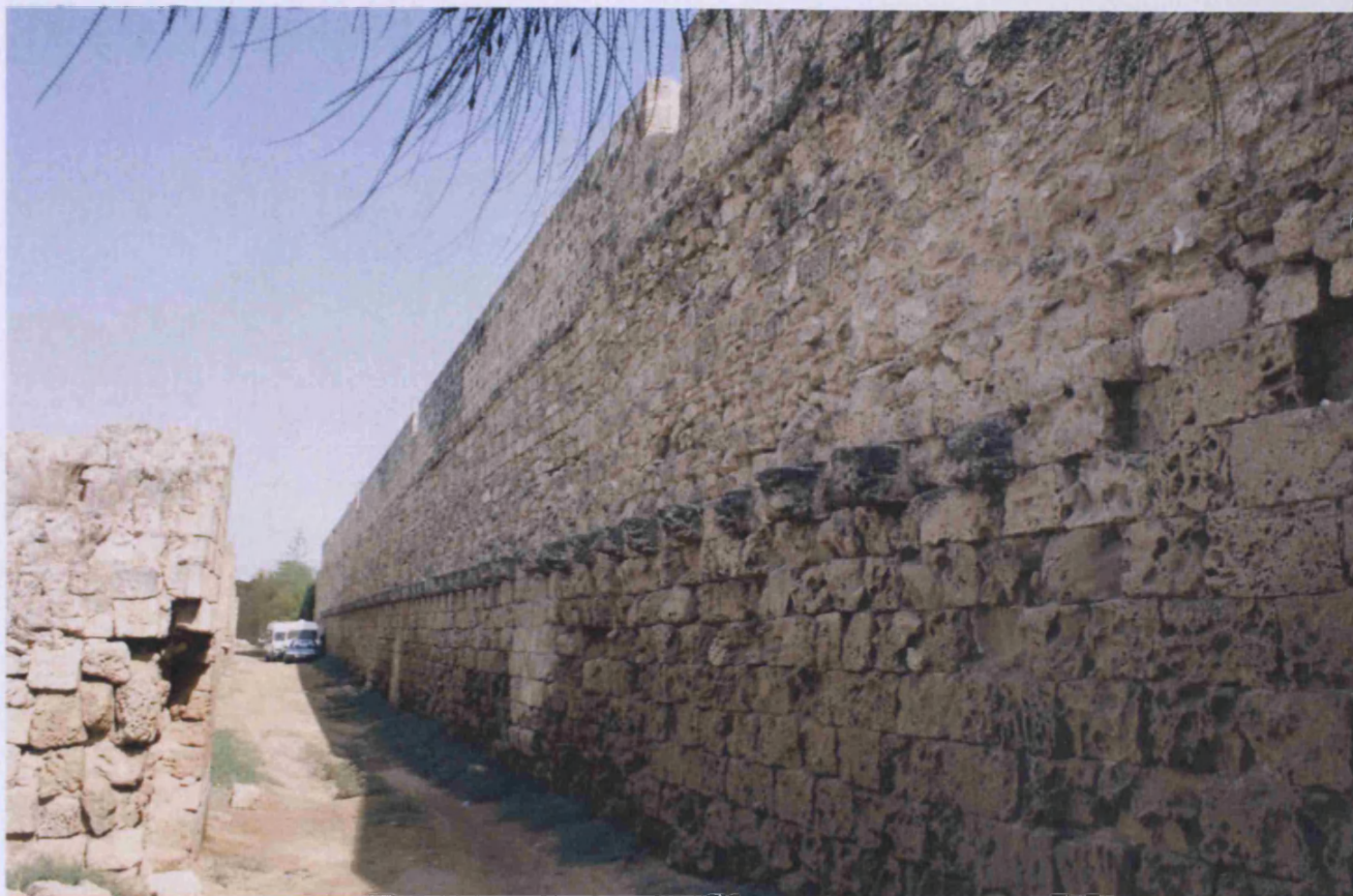
Interior of Lusignan wall running south from Venetian sea gate. The continuous line of corbels to carry a chemin de ronde is clearly seen. The uppermost (second storey) level with its embrasures for cannon is likely Venetian, as is the whole of the external facing of this sea wall.
