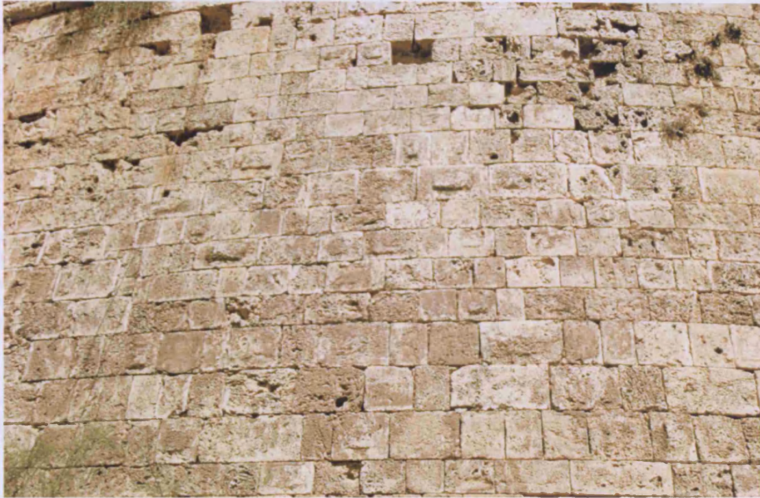
Detail of the exterior of the Arsenal tower showing occasional use of bossed masonry.
