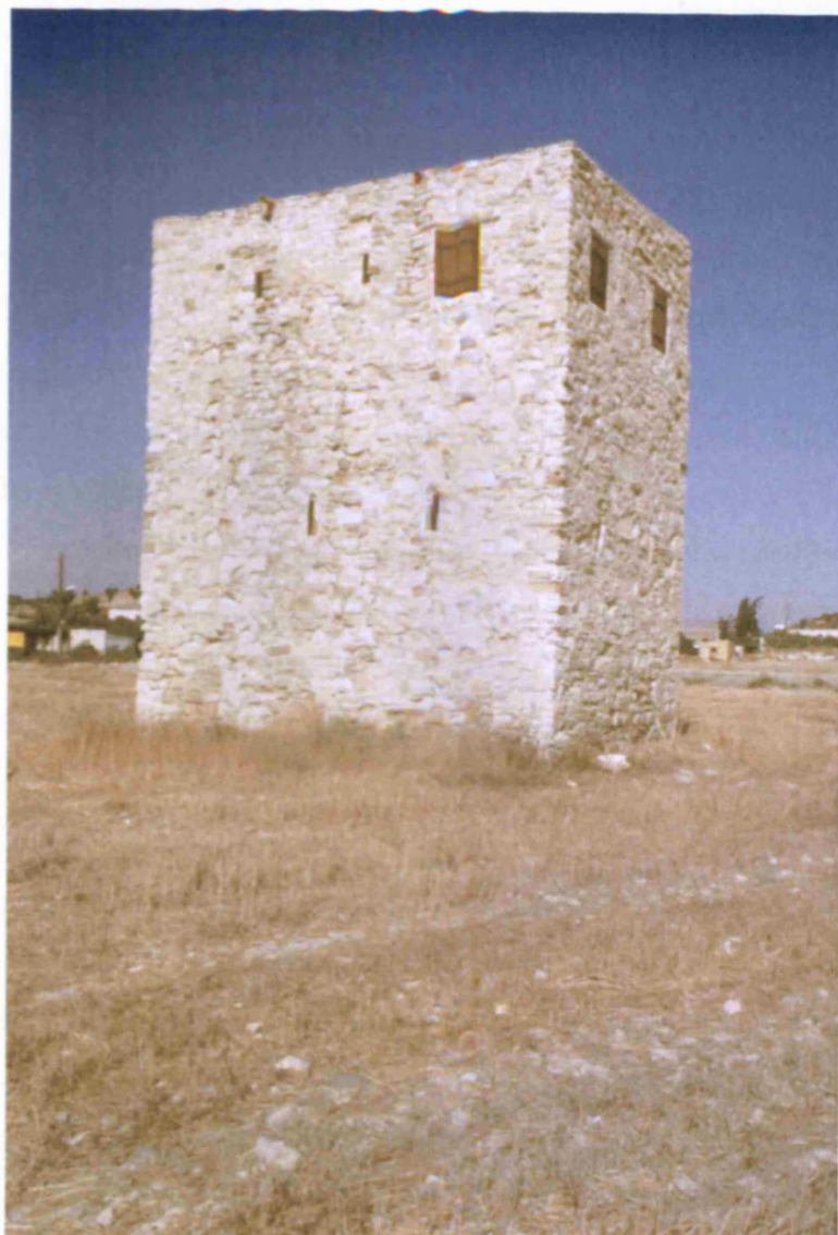
Rear face of tower.
