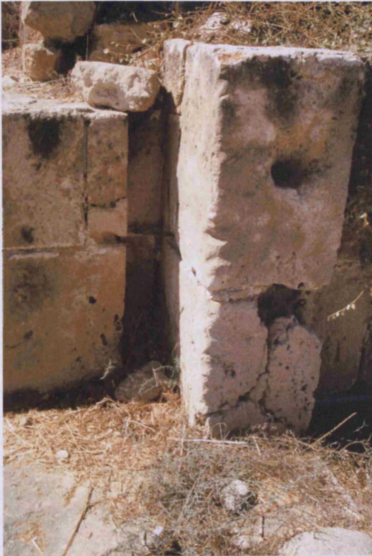
Portcullis groove on inner gatehouse (M on plan).
