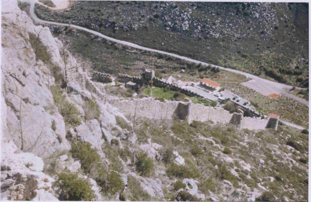
Lower ward/ bourg Byzantine curtain (6 on plan) with open backed semi-circular towers.
