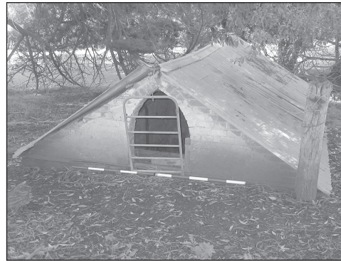
Figure 11.9 Stone water tank
