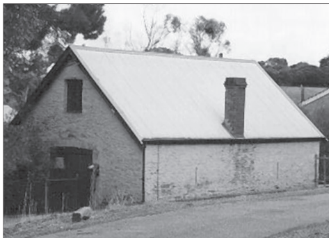
Figure 11.8 The Stone Barn, constructed between 1851 and 1858.
