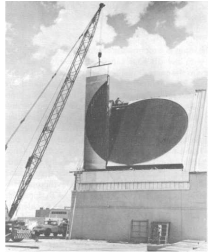
Figure 1.1: The HAPDAR is a phased array radar for tracking multiple airborne targets. The picture is from [6].
