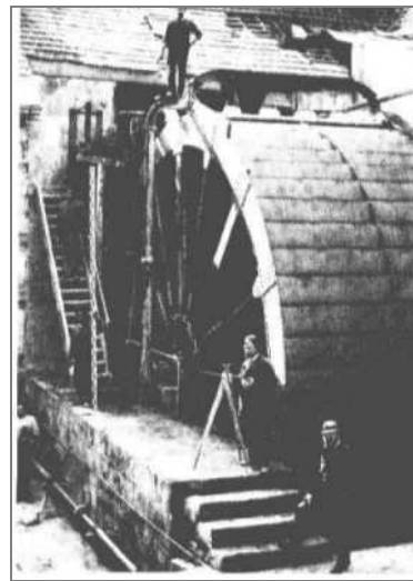
b. Overshot wheel 8.88m diameter, paper mill, Pfullingen / Southern Germany ca. 1900
