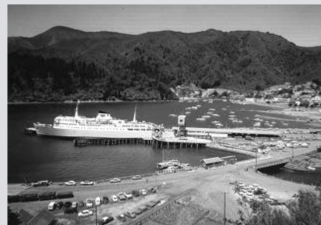
Above: Picton Harbour, with the roll-on, roll-off ferry Aramoana backed up to the linkspan, early 1960s.
