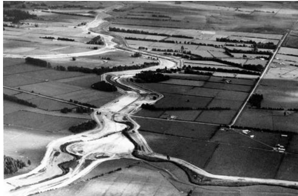
Above: This aerial view of a section of the Mangawara River control scheme depicts a series of stopbanks—a major aspect of the project. The sacrifice to farmland in terms of additional land being taken up between the banks is more than compensated for by the now certain relief from recurrences of the disastrous floods in the 1950s.
