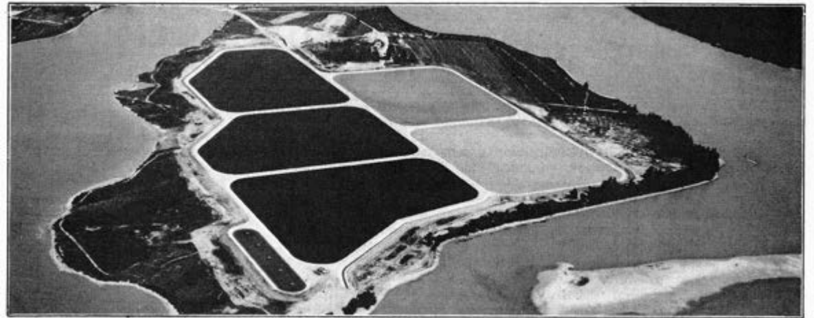
Above: The picture shows the oxidation ponds on Bells Island in the Waimea Estuary, part of the Nelson Regional Sewerage Scheme.
