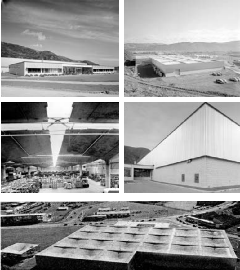
Above: The formwork for the shell units appears in the left foreground.
