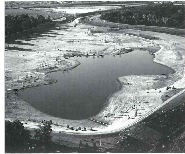
▲ Detention storage, such as this Mingo basin, can include amenities.
