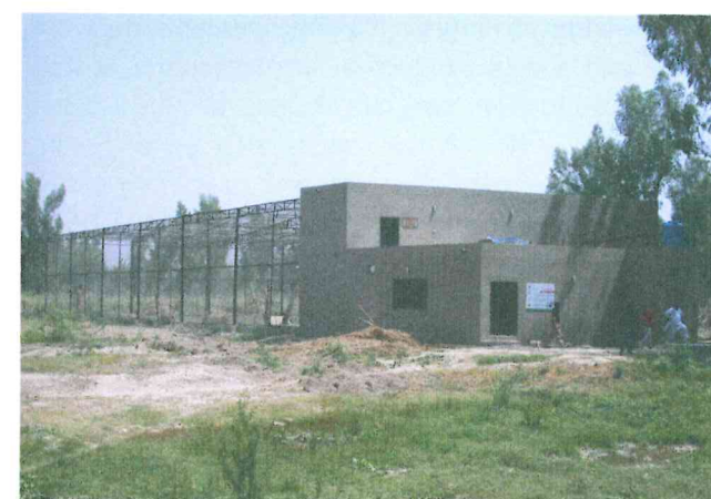
Fig. 3. Facility addition allowing for storage and office space.
