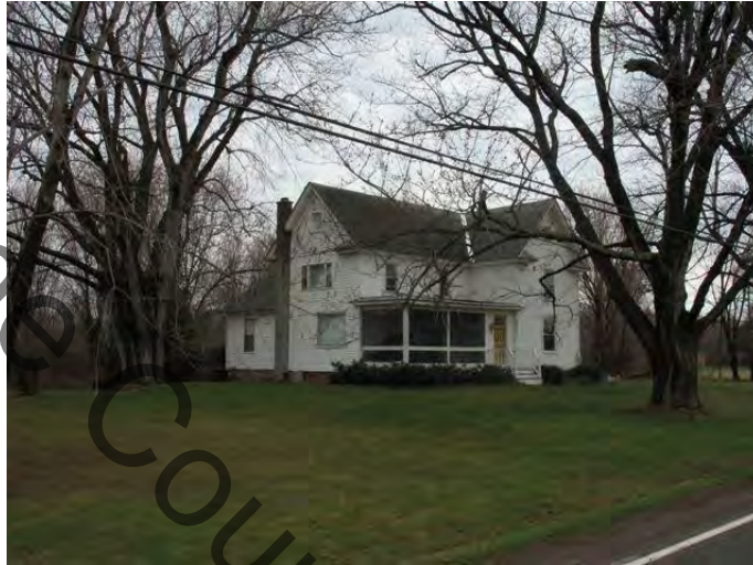
Site of Young home, looking west
