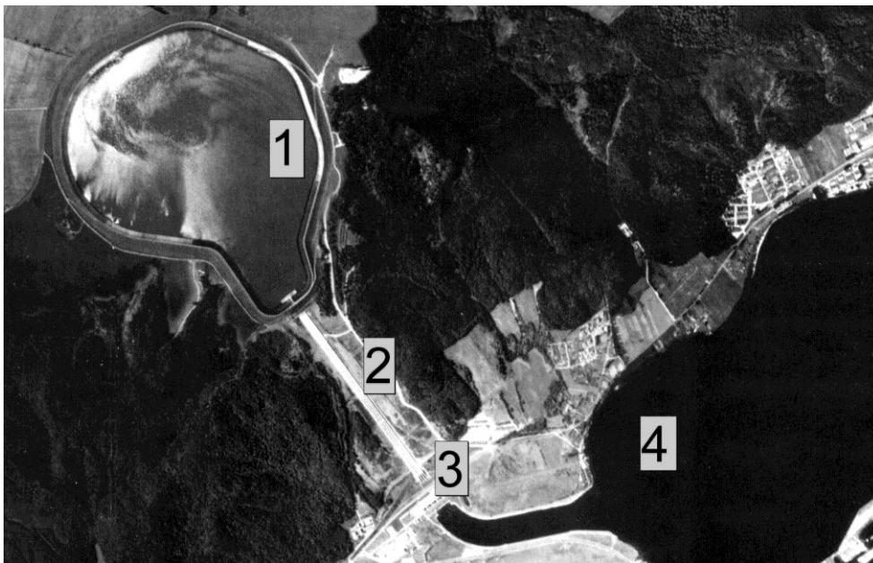
Fig. 1. Aerial view on the pumped storage power plant Zarnowiec (1-upper reservoir, 2- pipelines, 3-power plant building, 4-Zarnowieckie Lake).
