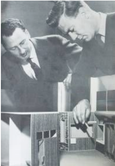
In 1963 work started on planning the rebuilding of the parts of the museum destroyed in the blitz.
