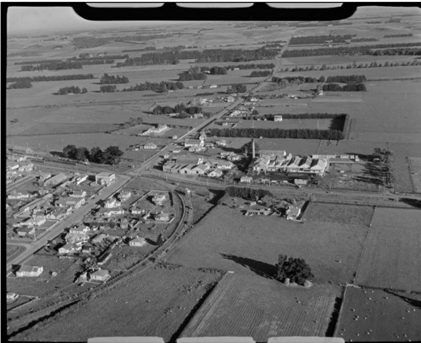
Figure 16. aerial view of the Edendale Dairy Factory in 1955 (Source: Client supplied image).
