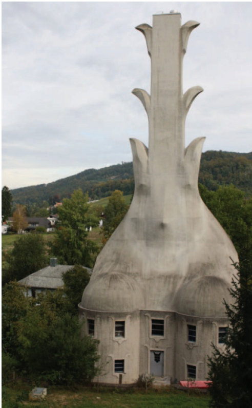
Figure 14. Boiler House, Rudolf Steiner. Photo: © Fiona Gray.
