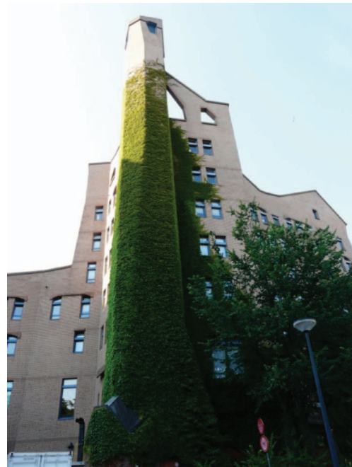
Figure 3. NMB Bank, Amsterdam, Ton Alberts and Max Van Huut, 1982. Source: http://commons.wikimedia.org/wiki/File:WLANL_-_jankie__ING_gebouw_Amsterdamse_Poort_(3).jpg . Licensed under the Creative Commons Attribution ShareAlike 2.0 License.
