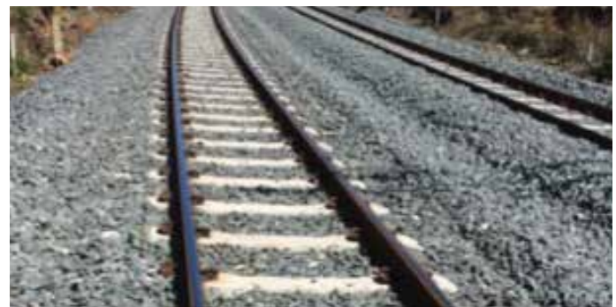
Figure 22: Example of track in good condition
