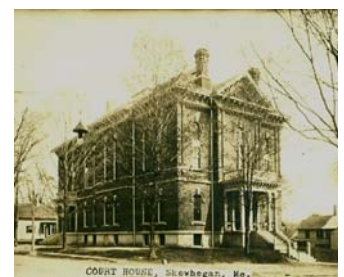
Somerset Court House ca. 1873
