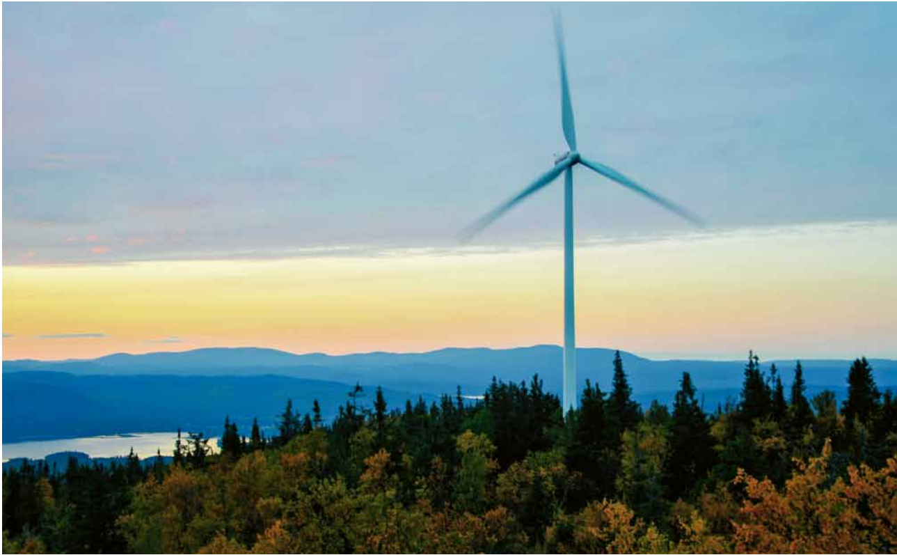
Sunset at Bleikevare wind farm with 18 wind turbines (36 MW).
