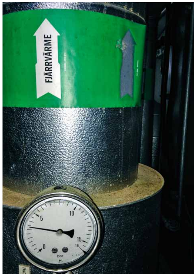
The district heating plant outside Helsingborg acquired by OX2 in 2013.
