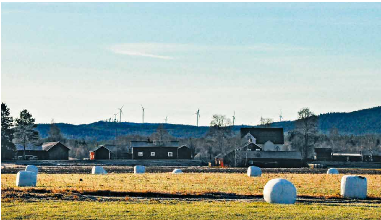
The 9-turbine Korpjället wind farm (20.7 MW).
