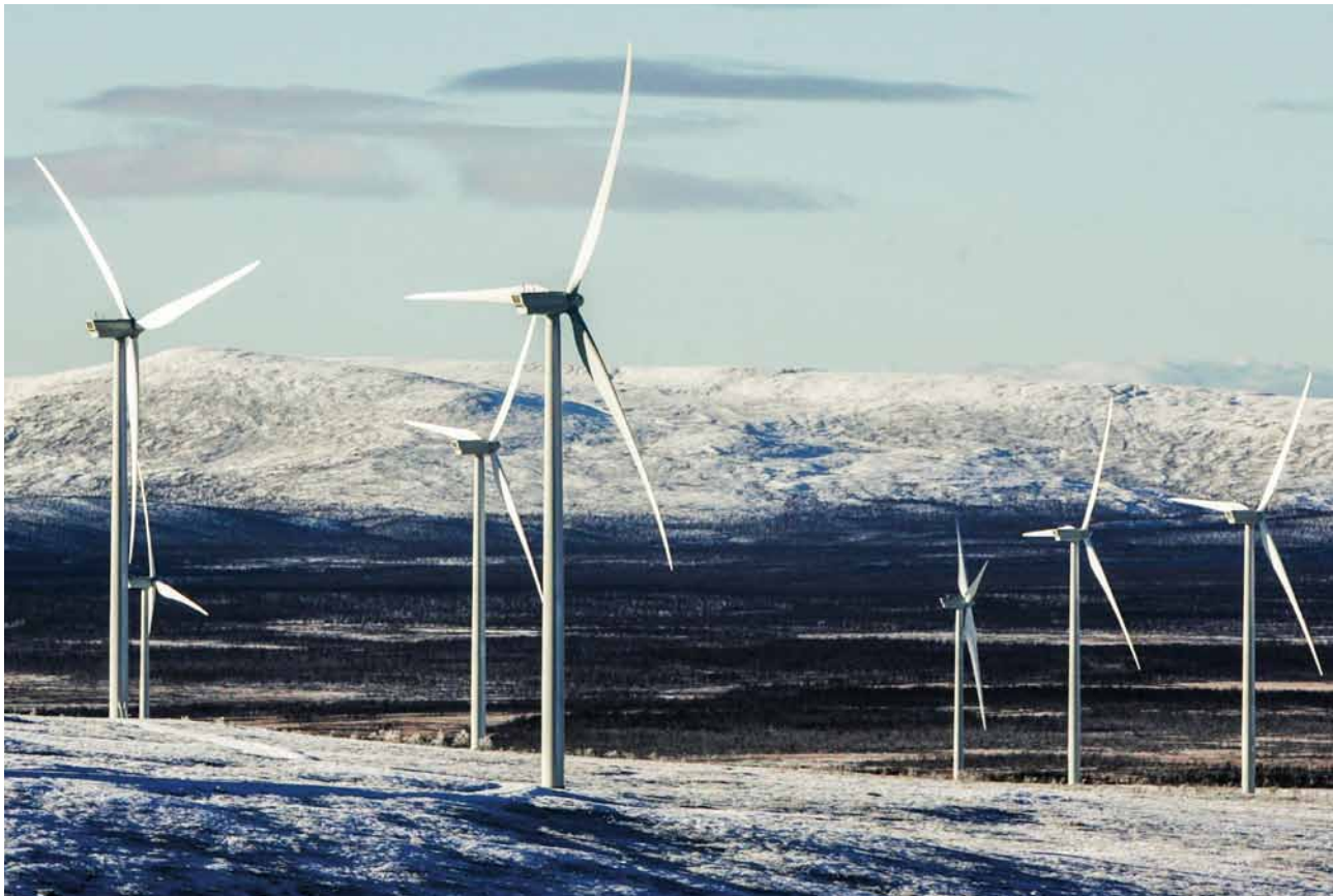
The Sjisjka wind farm with 30 turbines (78 MW) is owned by Skanska, OX2 and Jämtkraft. Photo: Kenneth Paulsson.
