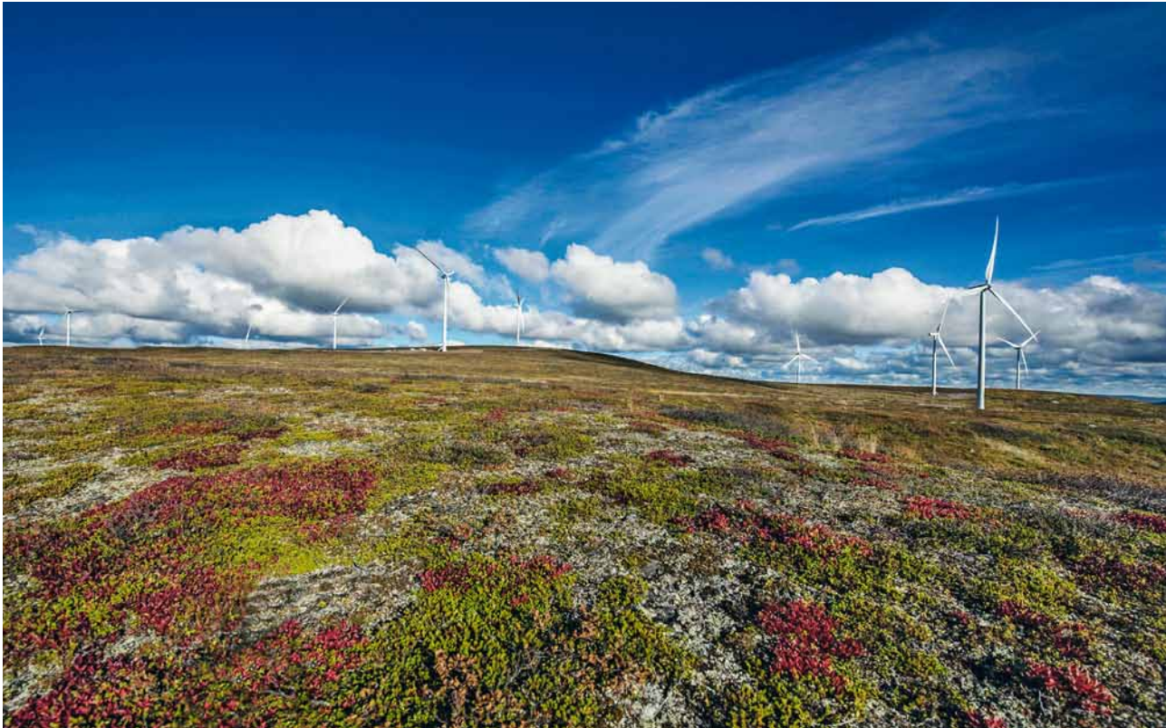
The Sjisjka wind farm in the Municipality of Gällivare is owned by Skanska, OX2 and Jämtkraft. In 2013, the farm produced 180 GWh.
