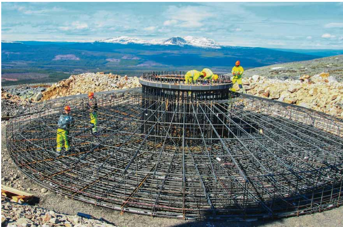
Reinforcement of wind turbine fundaments at Glötesvålen, Municipality of Härjedalen.
