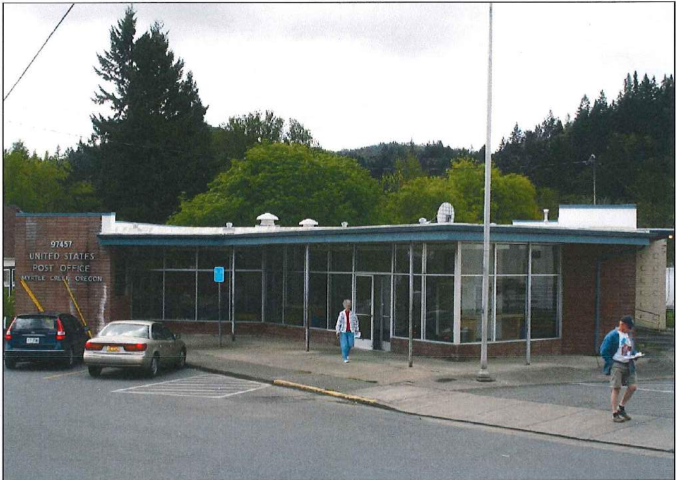
Figure 2: Myrtle Creek Main Post Office (124 Broadway Street, Myrtle Creek, Douglas County)
