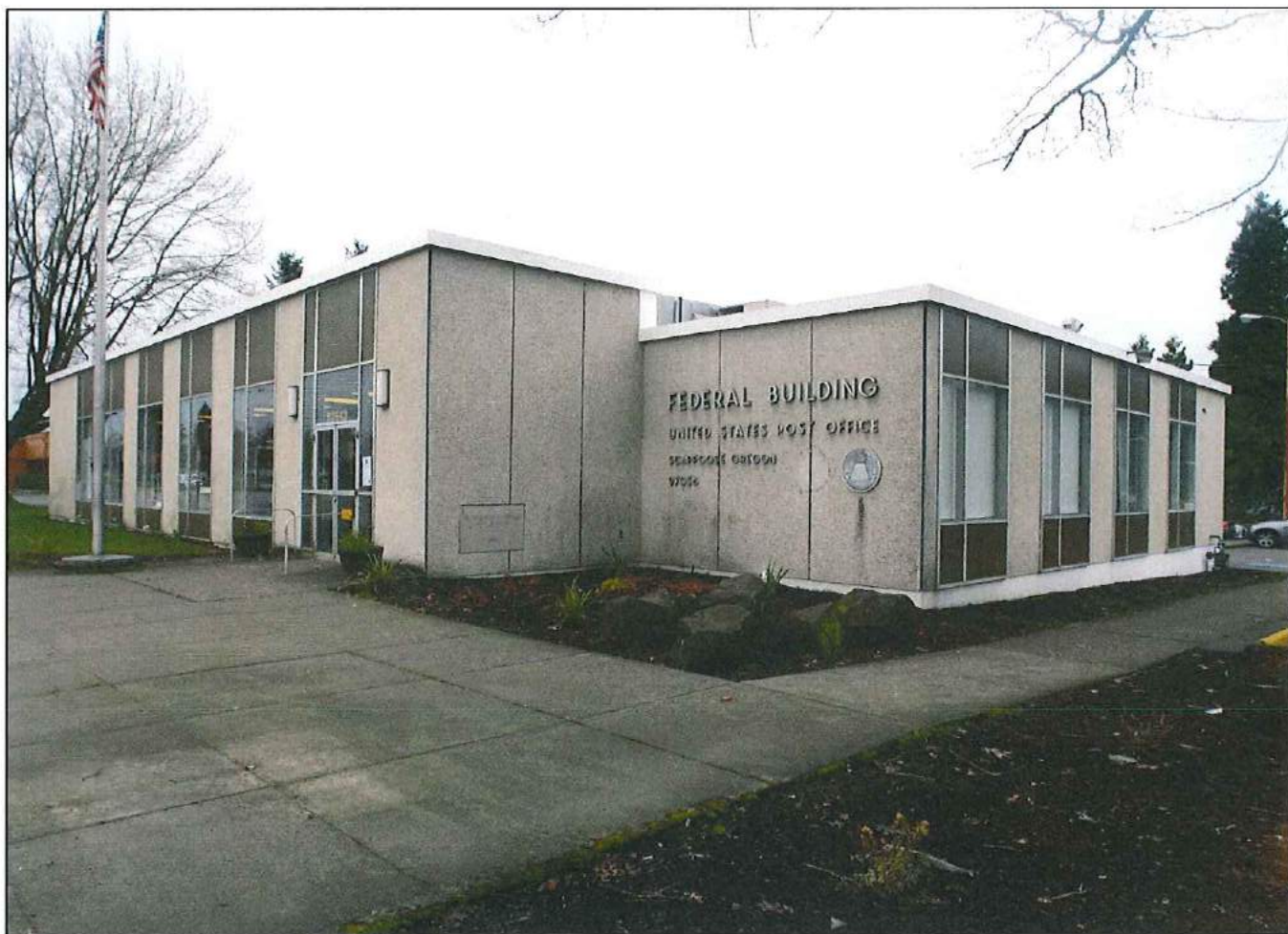
Figure 6: Scappoose Main Post Office (52643 Columbia River Highway, Scappoose, Columbia County)
