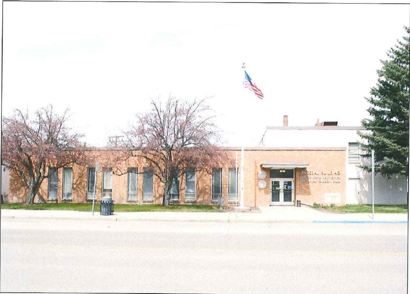
Figure 10: Federal Building/Post Office (201 W. North Street, Enterprise, Wallowa County)
